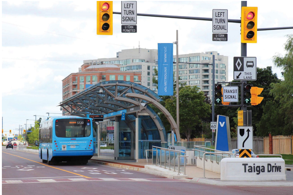
Figure 7-4: Bus-only Lane on Centre Street in Vaughan
