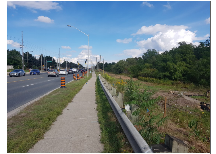
Rutherford Road recently cleared of vegetation
