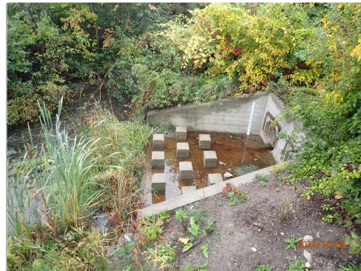
Plate 6: SWMP outlet into Don River West Branch.
