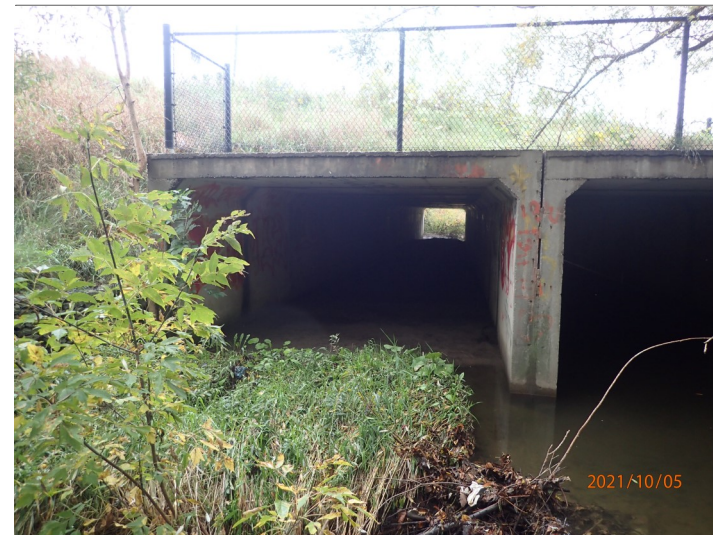
Plate 2: Culvert outlet at McNaughton Rd, facing upstream (north).
