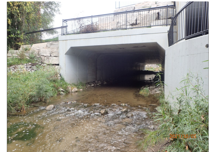
Plate 8: Major Mackenzie Drive culvert outlet, facing upstream (north).
