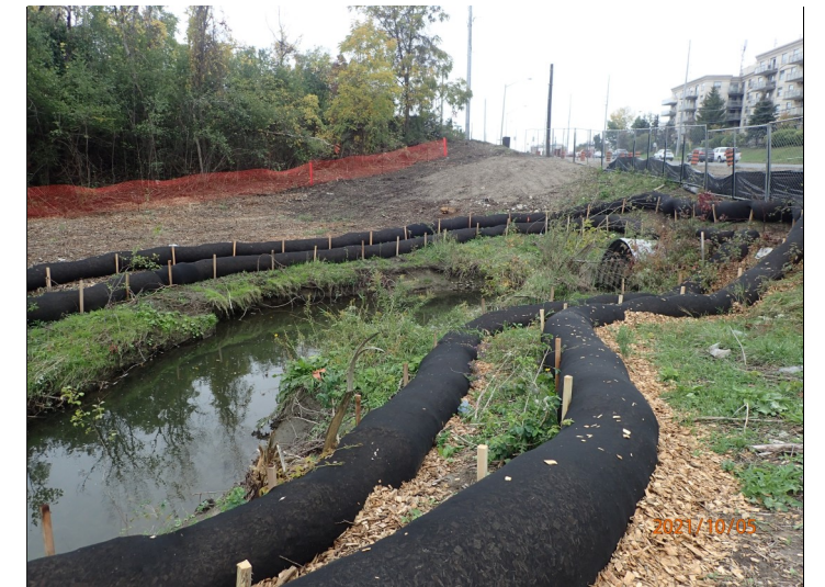
Plate 8: Rutherford Rd crossing, culvert outlet. Active works are occurring.
