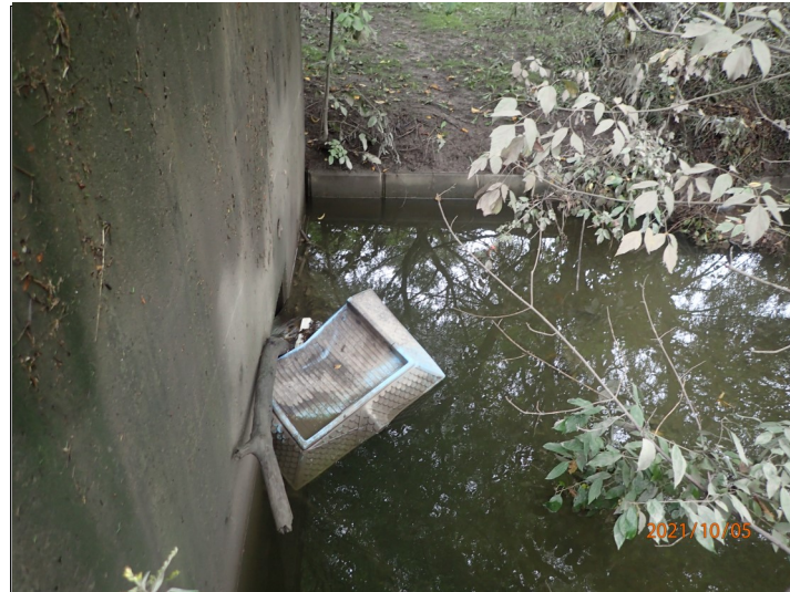
Plate 1: Proposed crossing over culvert, inlet.
