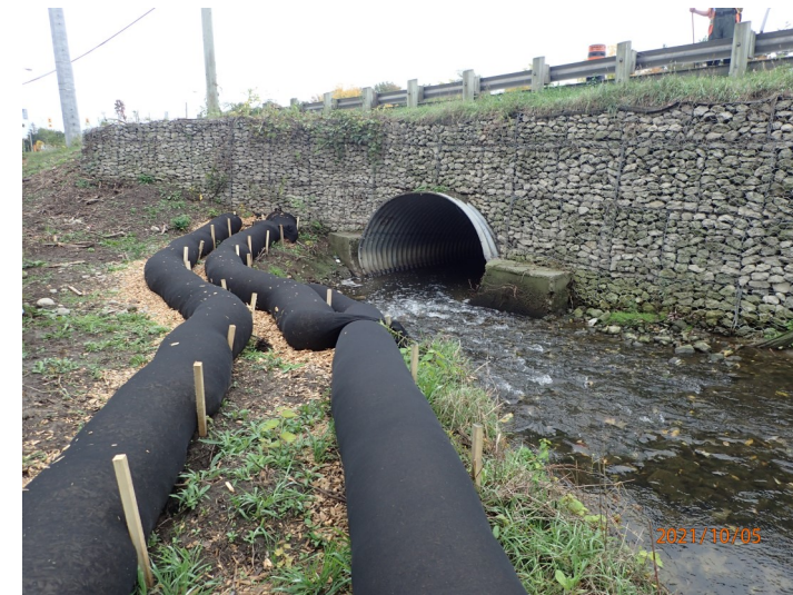
Plate 7: Rutherford Rd crossing, culvert inlet. Active works are occurring.
