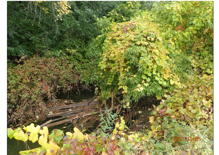
Plate 8: Partial debris jam at Bridge Crossing Option 3.
