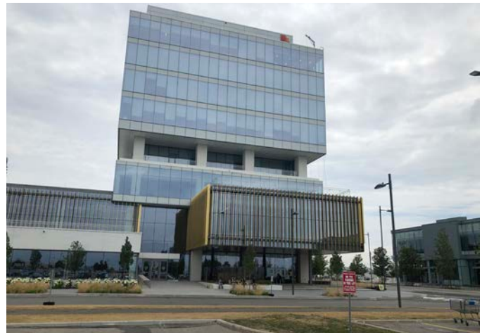
PwC office building with a YMCA and childcare, a public library, performing arts centre, a community kitchen, and ground floor retail
