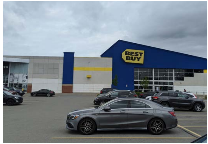
Large format retail north of Highway 7, west of Weston Road
