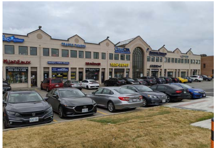
Retail commercial in La Piazza south of Highway 7, west of Weston Road
