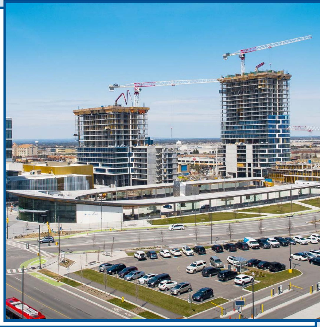
Vaughan Metropolitan Centre
