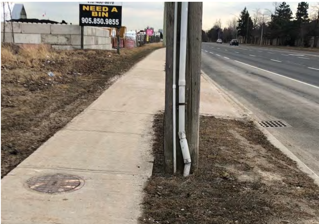
Catch basin and manhole observed along Weston Road in the vicinity of Weston Road and Astona Boulevard intersection.
