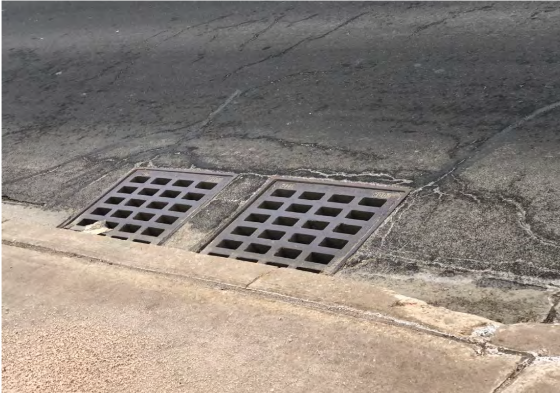
Catch basins observed along Weston Road.
