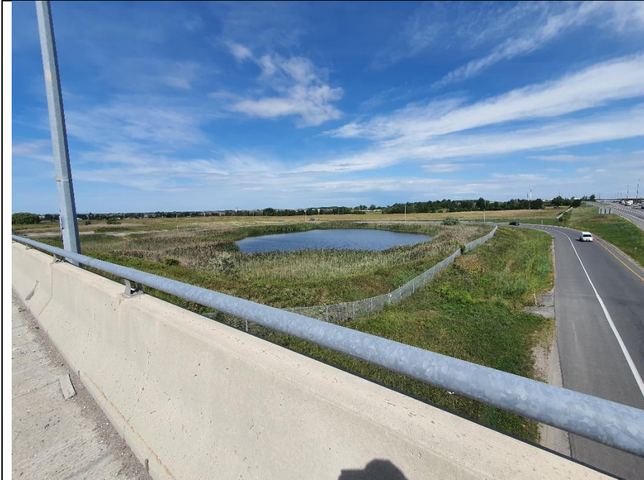
Photo of the ramp entrance to highway 400. Pond was observed in the middle of the ramp. The photo was taken facing Northwest direction.
