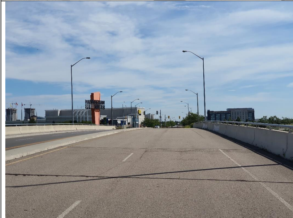
Photo of Fishermens Way, taken from Bass Pro Mills Drive, near the ramp entrance to highway 400. Photo was taken facing East
