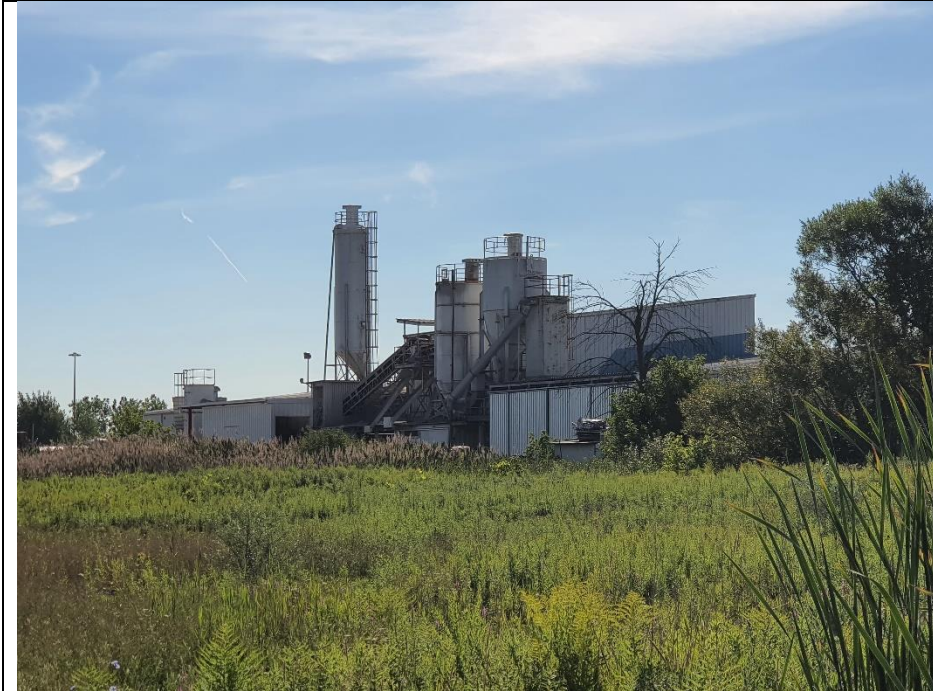
Photo of the plant behind Best Way Stone. Likely used as stone slab/ concrete manufacturing plant, as reported in ERIS report. The photo was taken facing Southeast.
