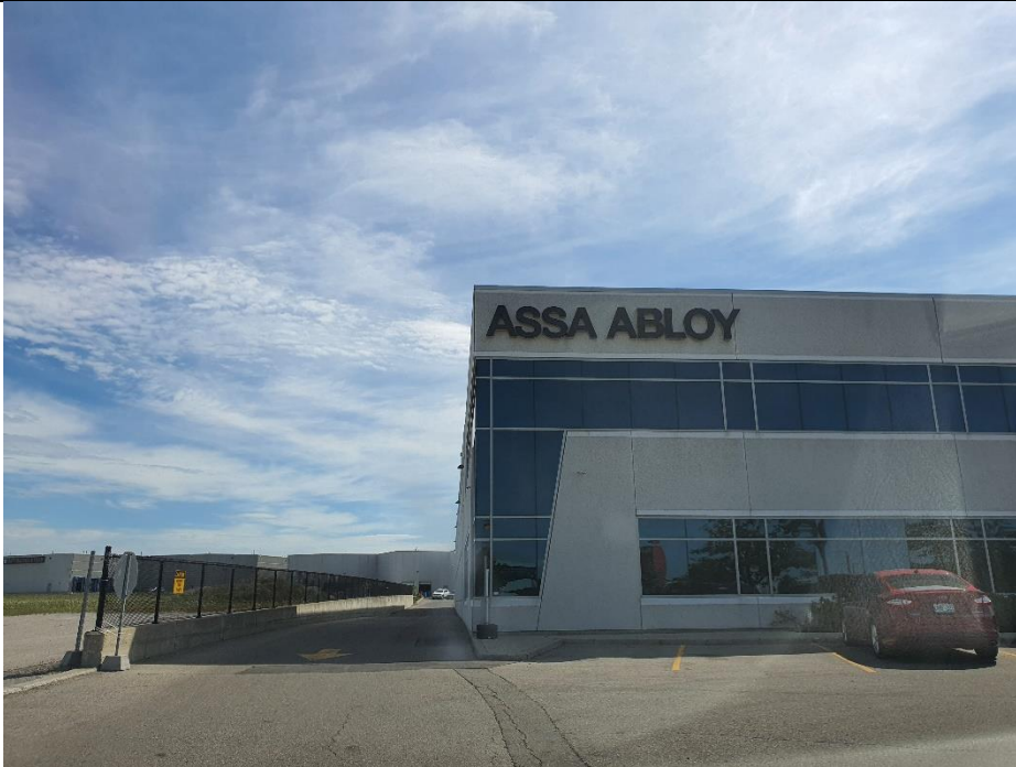
Photo of ASSA ABLOY, located at 160 Four Valley Drive, just east of Miele. Found to previously be a manufacturer of various machinery, electronics and hardware products. Photo taken facing east.
