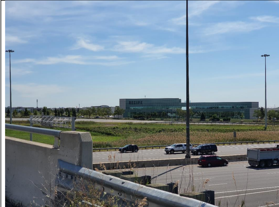
Photo of RECIPE building, located at 199 Four Valley Drive, at the Southwest corner of the Site boundary, and highway 400. Photo was taken facing Southwest.
