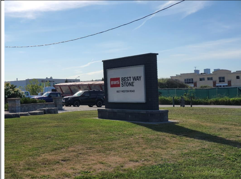
Photo of Best Way Stone, a stone distribution and likely manufacturing facility. Reported through ERIS as concrete manufacturing facility. Photo was taken facing Southeast.
