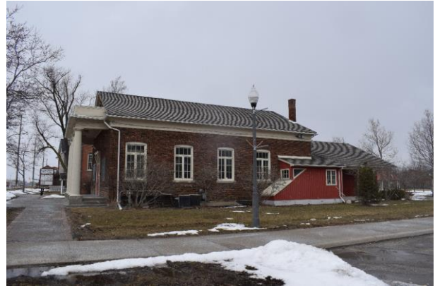
Plate 2: 9541 Weston Road looking north
