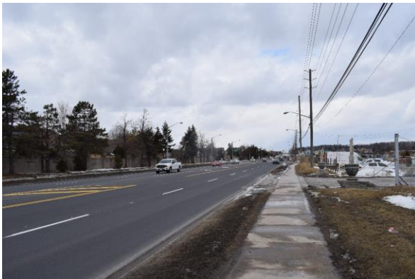
Plate 3: Weston Road looking north
