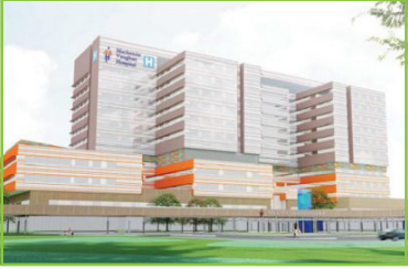
// Future Mackenzie Vaughan Hospital
