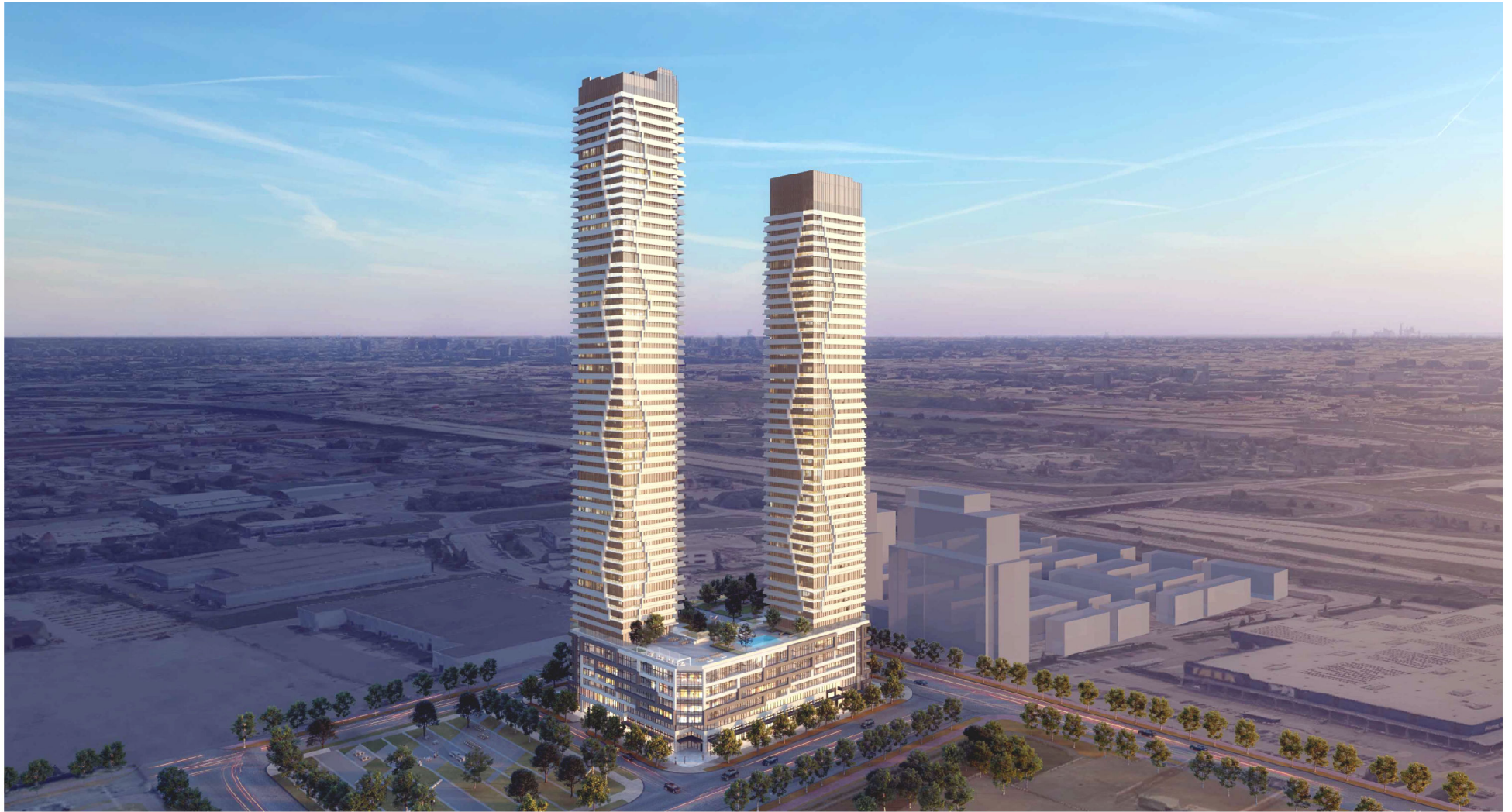
VIEW LOOKING SOUTH-EAST
