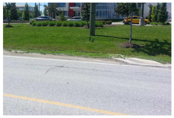
Photo 13: Slight to moderate wheel track rutting and cracking
