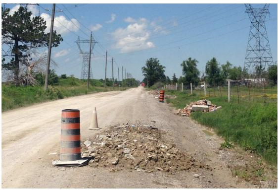
Photo 20: Improper construction debris disposal and no proper ditching along the road
