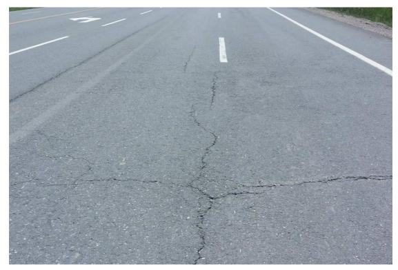
Photo 4: Slight to moderate transverse cracking
