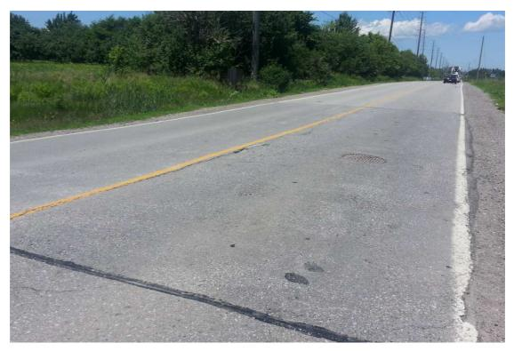
Photo 9: Slight to moderate raveling and coarse aggregate loss with potholes
