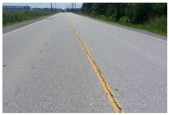
Photo 7: Slight to moderate longitudinal construction joint
