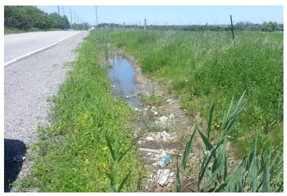
Photo 8: Standing water and dumped garbage at northbound ditch
