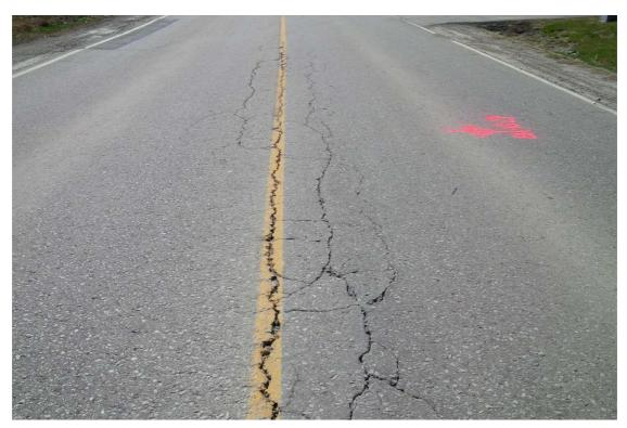
Photo 11: Slight to severe multiple centerline cracking
