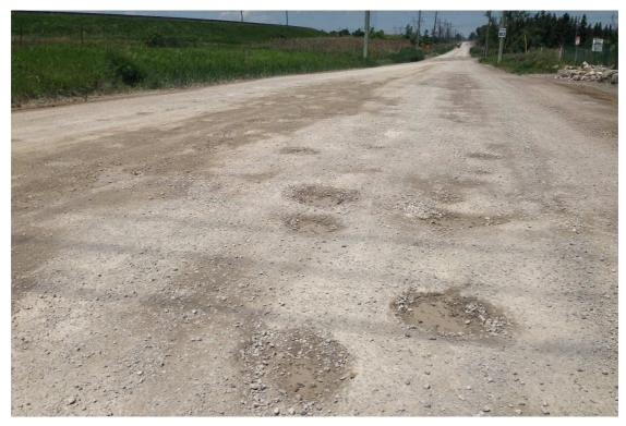
Photo 17: Potholes/waterponds and uneven surface of the gravelly road
