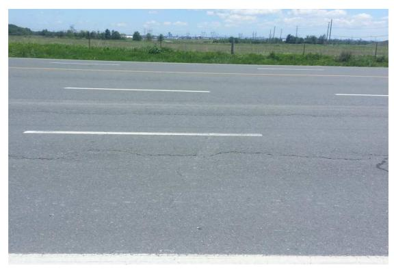
Photo 3: Slight to moderate wheel track rutting and cracking
