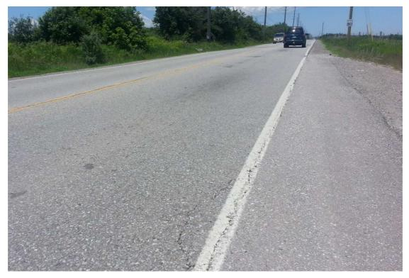
Photo 6: Slight to moderate pavement edge cracking and flushing
