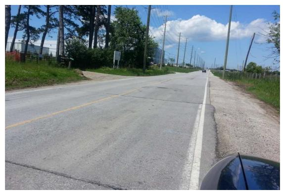
Photo 15: Uneven surface of the road and no proper ditching
