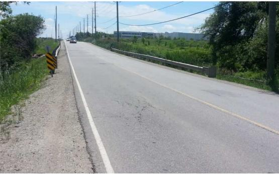
Photo 14: Slight to moderate map cracking and uneven surface of the road
