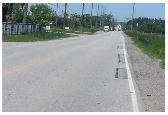
Photo 10: Patching along pavement edge of the road
