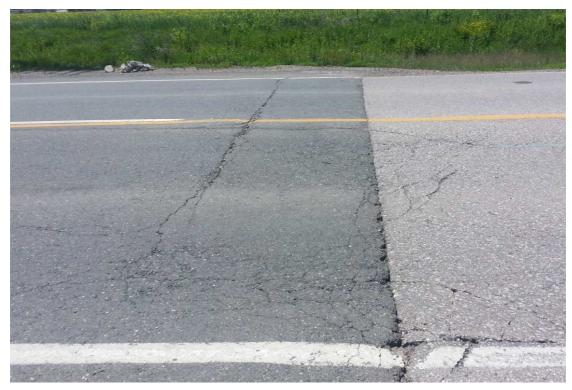
Photo 5: Slight to moderate transverse construction joint, moderate to severe transverse cracking, slight to moderate alligator cracking with potholes
