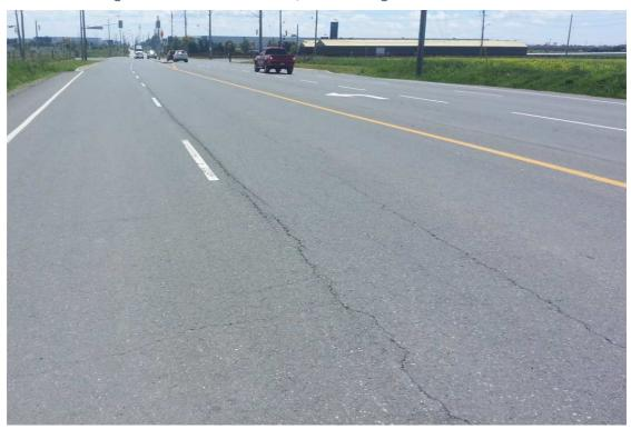
Photo 2: Slight to moderate longitudinal construction joint and midlane cracking
