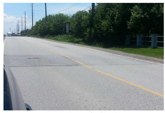
Photo 12: Patching around manhole and uneven surface of the road
