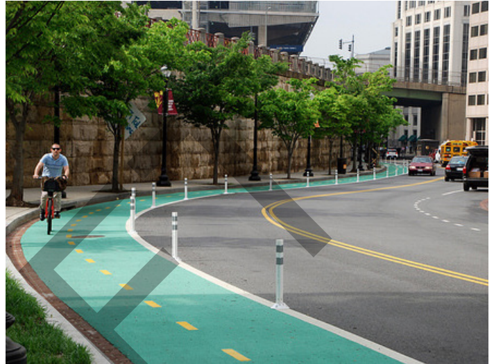
Figure 23. Protected bike lane in Washington DC source: www.ggwash.org
