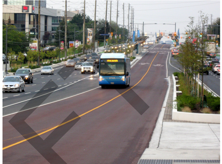
Figure 21. Highway 7 Bus Rapid Transit Corridor, Toronto source: Spacing Magazine
