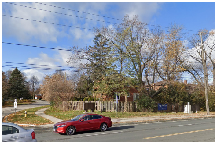
Figure 11. North Area - residential homes backlotted onto Yonge Street
