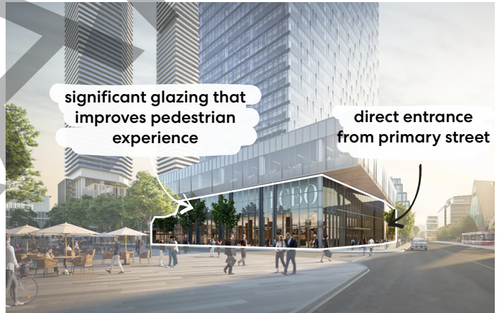
Figure 43. Ground floor retail at 100 Queens Quay East, Toronto source: www.plangroup.ca
