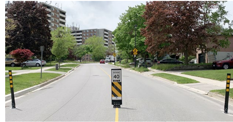
Centreline Bollards / Flex Bollards
