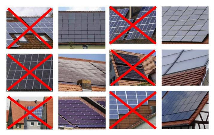
Image 63. Comparison between acceptable and not-acceptable integration of PV systems over traditional clay-based roof systems<sup>38</sup>
