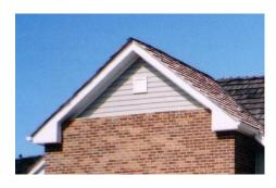
Image 26. Incorrect pre-finished metal 'box' termination
