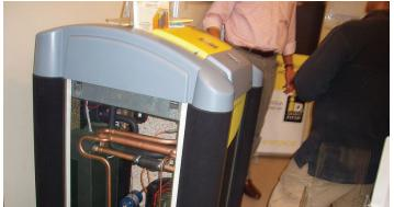
**Ground Source Heat Pumps (Geothermal)** A ground source heat pump (GSHP) works by utilizing the stable temperatures of the ground to reject heat in the summer and extract heat from in the winter.
