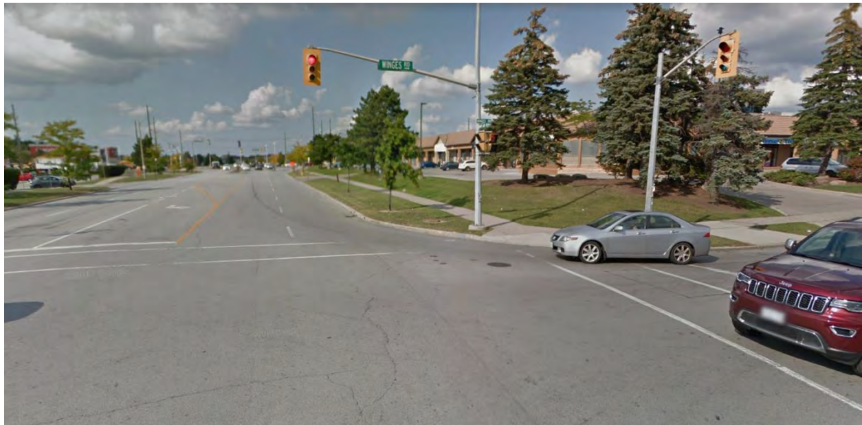
Figure 3-28. Large Turning Radii at the Northeast Corner of Whitmore Road and Wings Road
