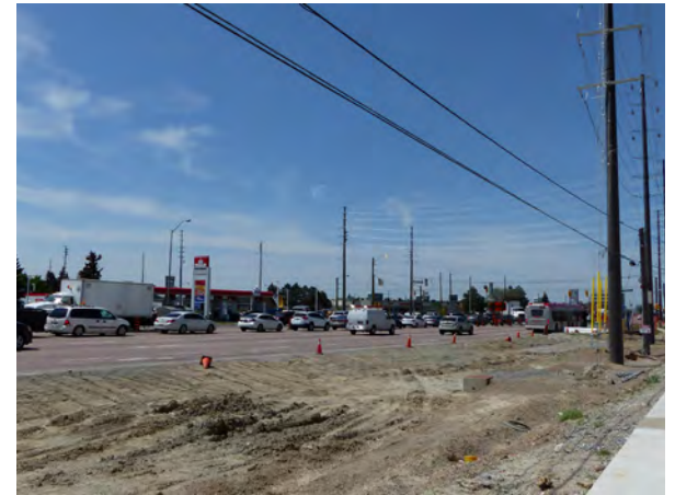
Road Work along the Highway 7 rapidway
