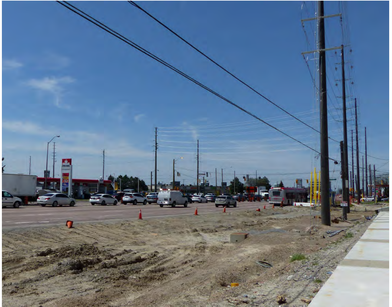
Highway 7 Rapidway construction today
