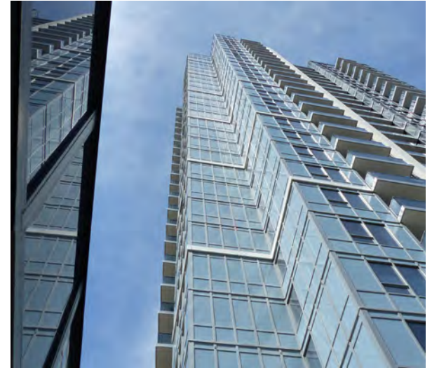
Centro towers are 30 and 33 storeys in height
