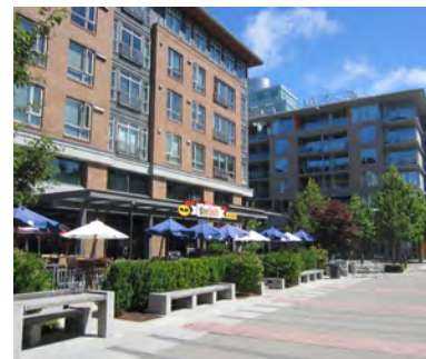
Mid-Rise Mixed Use Areas: Wesbrook Mall, Vancouver, British Columbia
