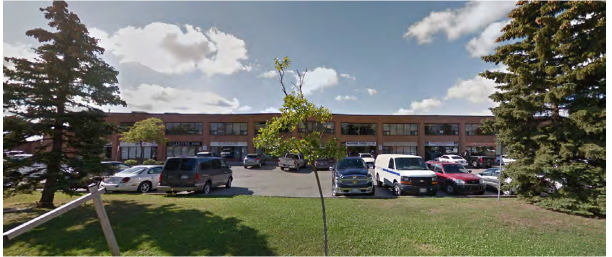
Designated employment lands about the Weston 7 SPA along the south side of Wings Road
