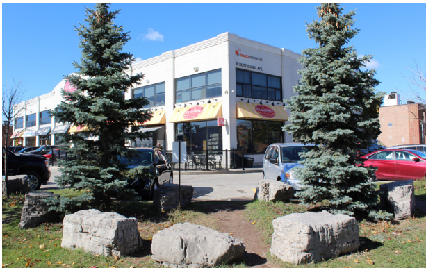
Image 8 Immediately north of the VMC are retail/service commercial uses
