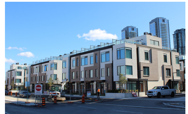
Image 16 Townhouses in the northeast quadrant
