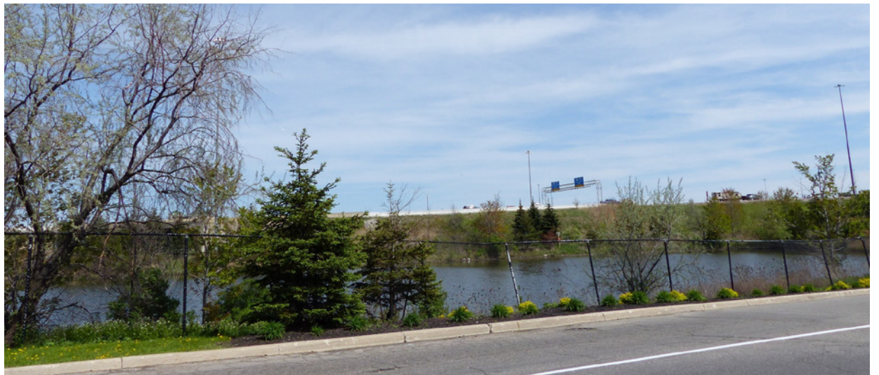
An engineered stormwater management pond south of Colossus Drive abuts the Highway 400 Corridor
