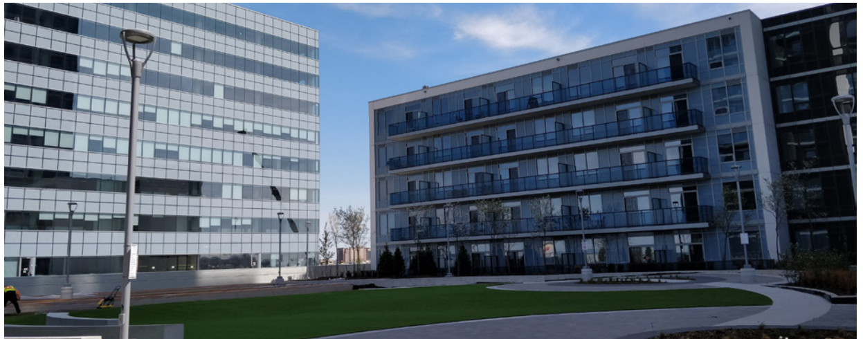
A 10 storey office component to the Centro development fronts Northview Blvd.
