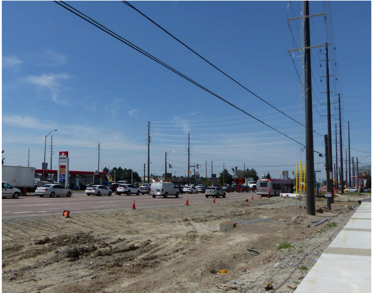
Highway 7 Rapidway construction today
