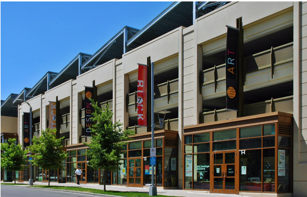
A parking garage in Belmar, Denver, Colorado, features retail storefronts at the ground floor and solar panels on the upper level (Source: sitephocus.com).
