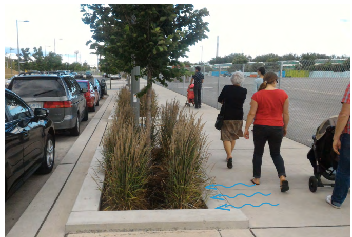
Planter edge open on one end, and sidewalk graded towards it for rain capture.
