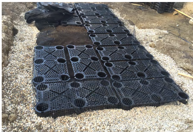
Use of a soil cell system provides extra support for greater compaction of hard surfacing of sidewalks, to protect the soil medium for healthy tree growth.
