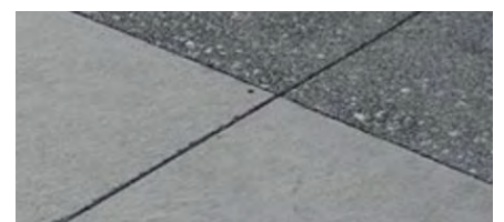
Concrete parking and sidewalk areas varying in finish, and incorporating a roll curb.
