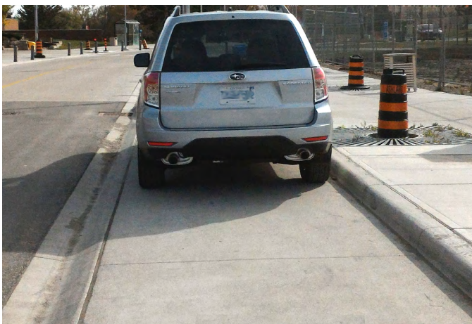
On-street parking with mountable curb.
