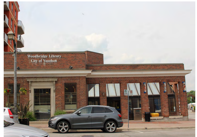
150 Woodbridge Avenue Woodbridge Public Library (1992)
