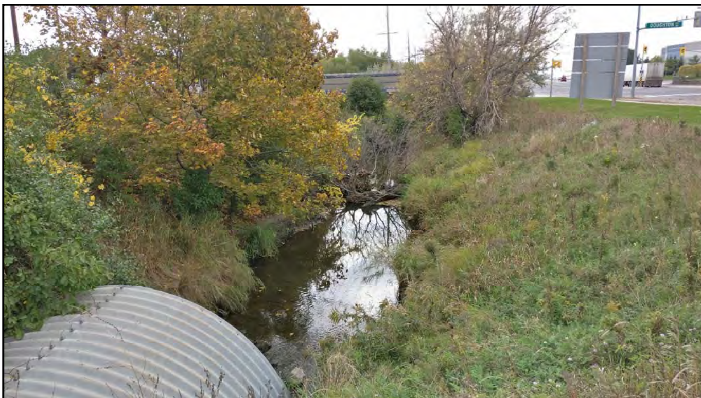
Black Creek Channel Culvert at Highway 7 looking south
