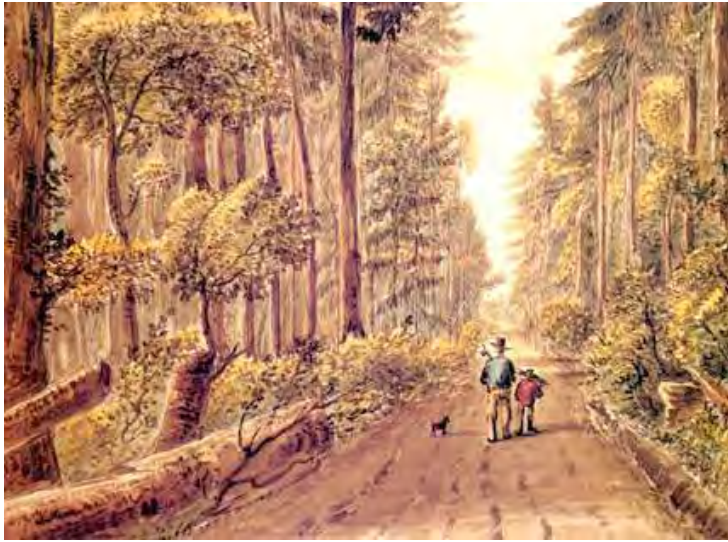
Under the Statute of Labour, clearing and maintaining the early roads was the responsibility of the land owners adjacent
