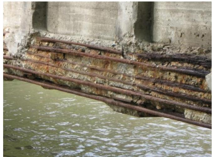
Figure 4. Truss Bottom Chord Showing Severe Spalling
