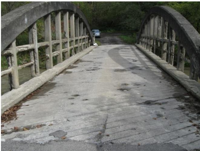
Figure 3. Bridge Deck Showing Cracks and Potholes
