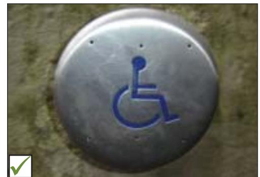
*Large circular power door operator control, clearly marked with International Symbol of Accessibility.*
