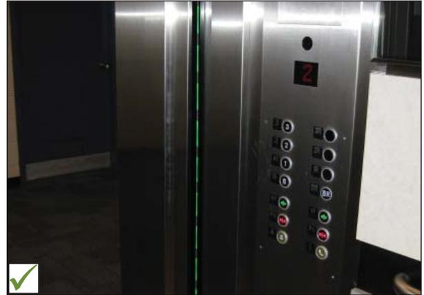
*Elevator sensor door and floor registration buttons.*
