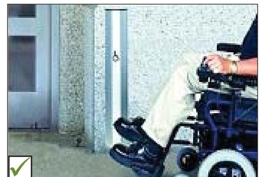
*Long extended power door operator control can accommodate a wider range of users (e.g., can be operated by foot or foot rest).*
