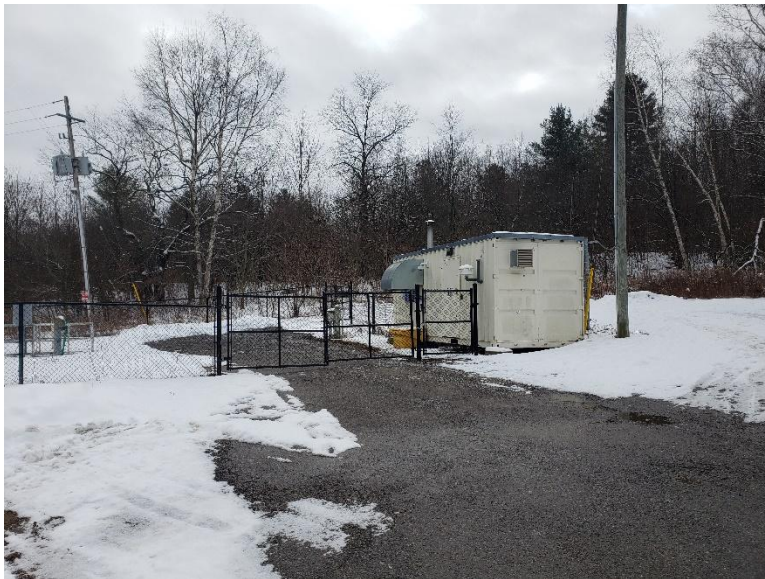
Figure 57: Fenced-off maintenance area for adjacent stormwater pond (A.S.I., 2025)
