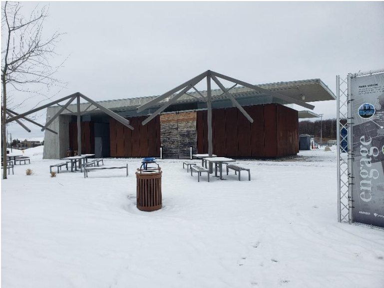
Figure 31: Picnic area on south side of pavilion, looking north (A.S.I., 2025)
