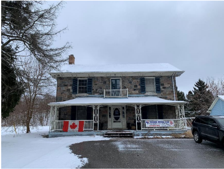
Figure 16: Front (west) façade of the Vaughan Soccer Club headquarters at 11151 Keele Street (A.S.I., 2025)
