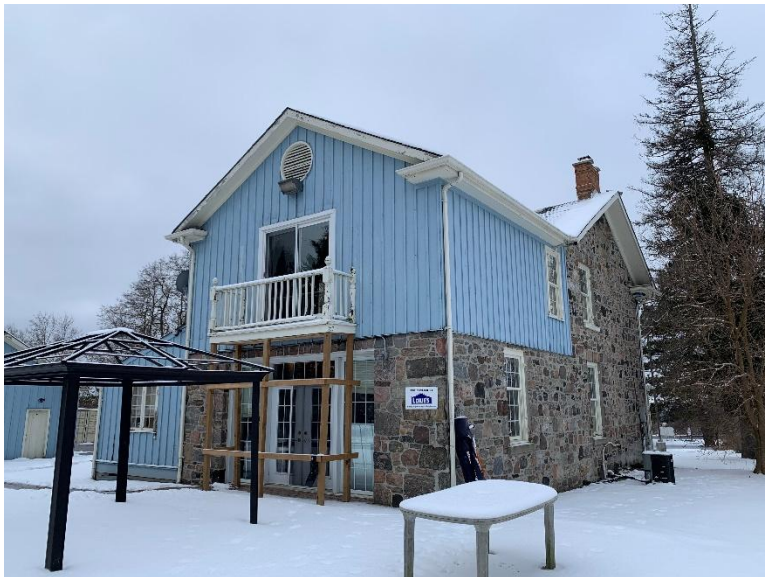
Figure 19: Addition to the east façade of the Vaughan Soccer Club headquarters, looking southwest (A.S.I., 2025)
