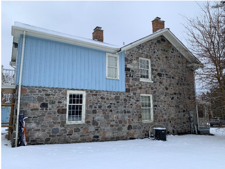
Figure 20: Rubble stone exterior on the north façade of the Vaughan Soccer Club headquarters (A.S.I., 2025)
