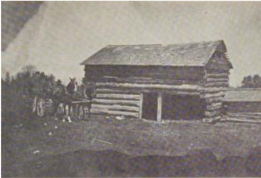
Figure 90: Log structure on Dufferin Street, Concession 3, north of Maple Sideroad (now Major Mackenzie Drive), date unknown (Reaman, 1971)
