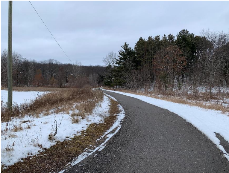
Figure 52: Paved pathway, looking northwest (A.S.I., 2025)
