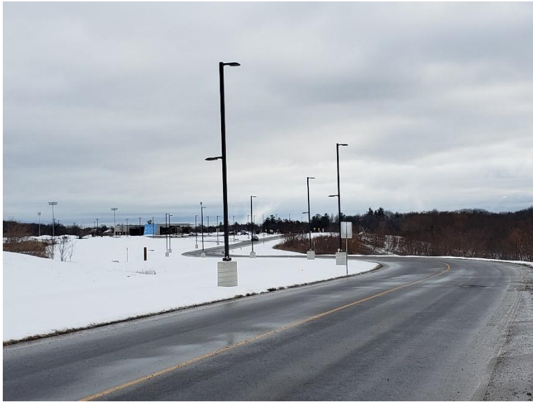
Figure 28: Vaughan CARES Way, looking east to pavilion building (A.S.I., 2025)
