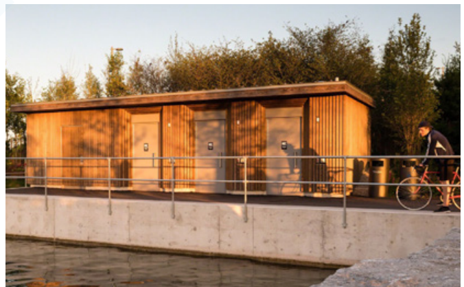
Trillium Park washrooms
