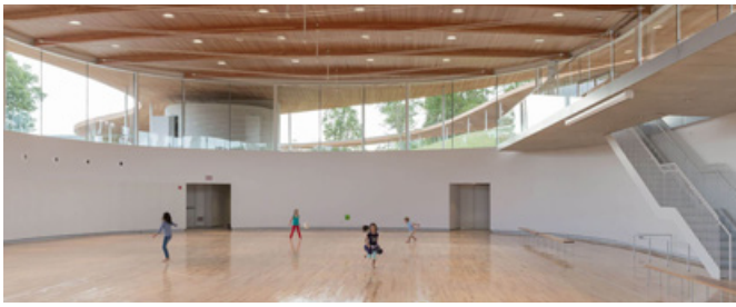
Grace farms indoor courts
