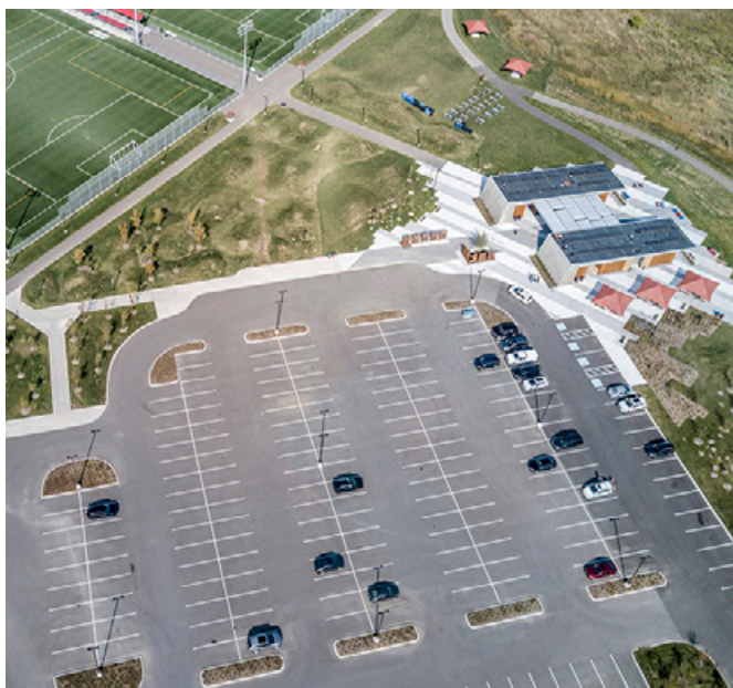
Drone photograph of existing pavilion and parking lot
