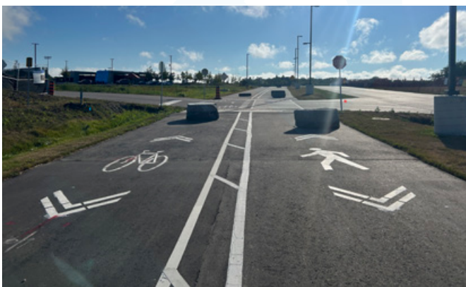
Active transportation network at Vaughan CARES Way
