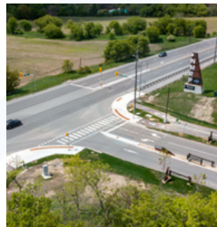
Keele Street Intersection aerial
