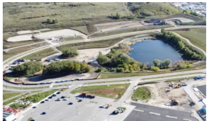
Pondsides District under construction (2025)
