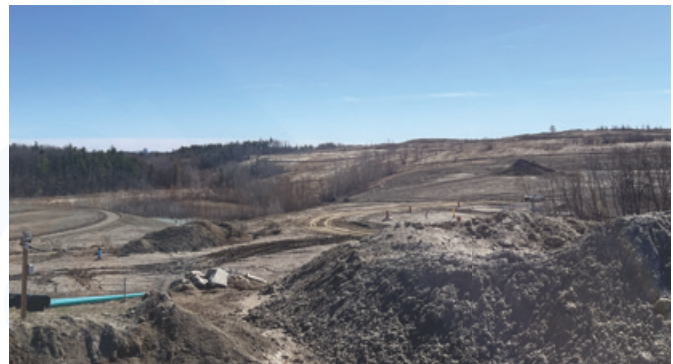
Enabling works construction (2024)
