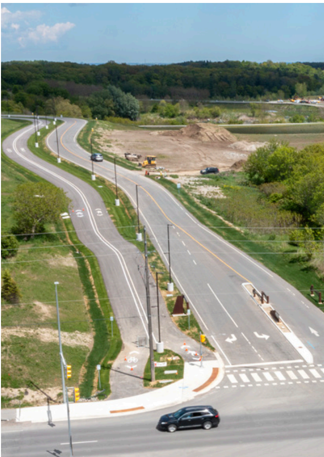
View into the park from Keele Street
