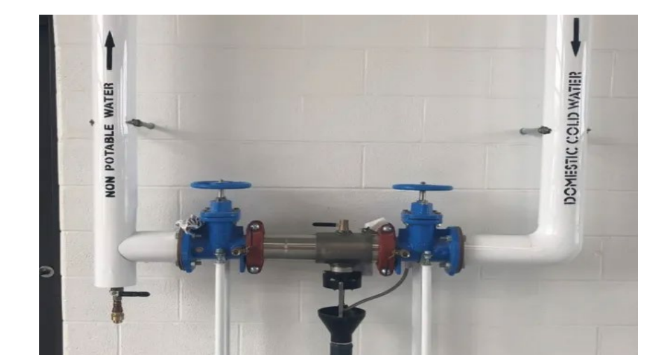
Water pipes with backflow prevention device
