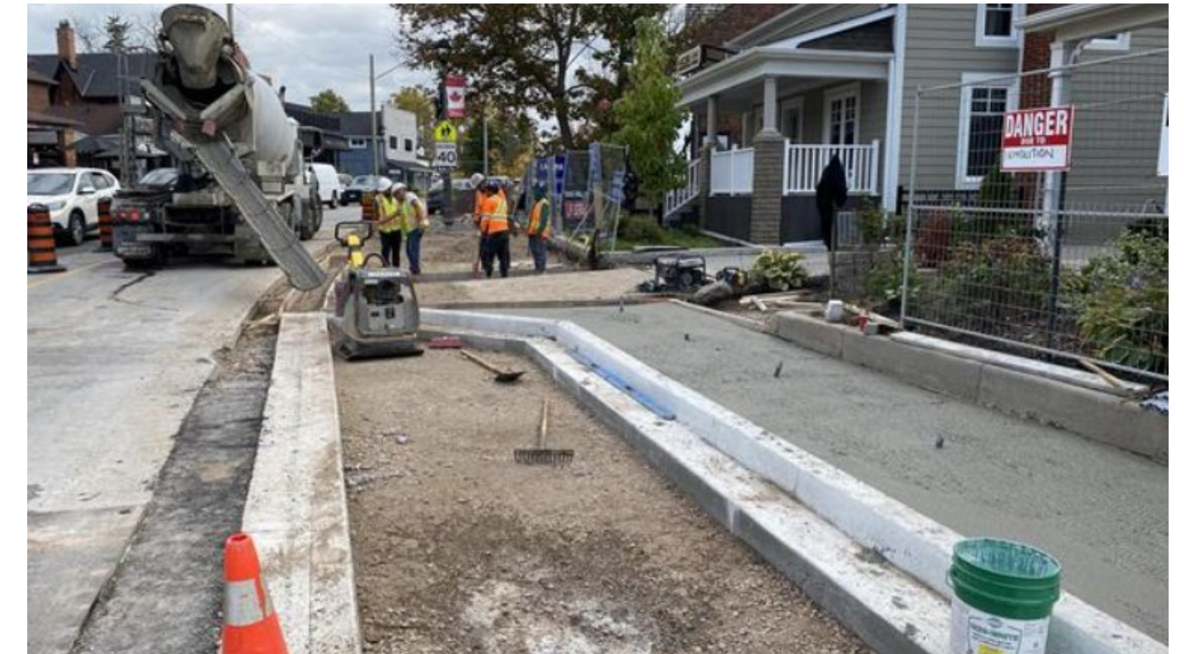
Typical streetscaping construction of curb, lay-by parking and sidewalk
