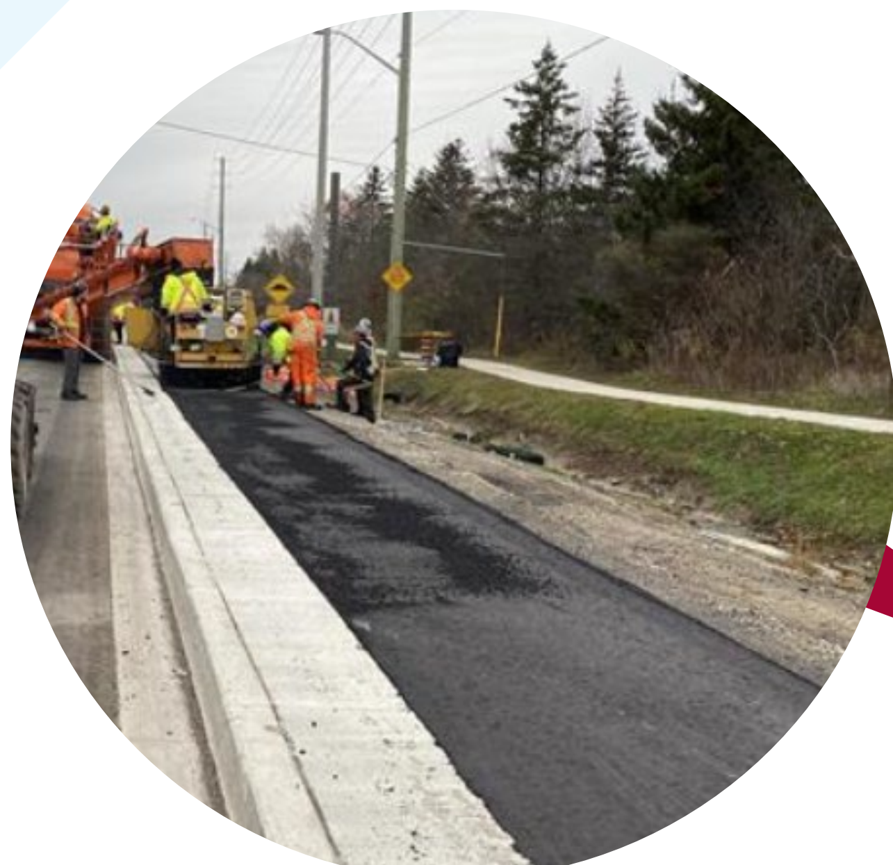
Cycling paths under construction on both sides of Islington Avenue
