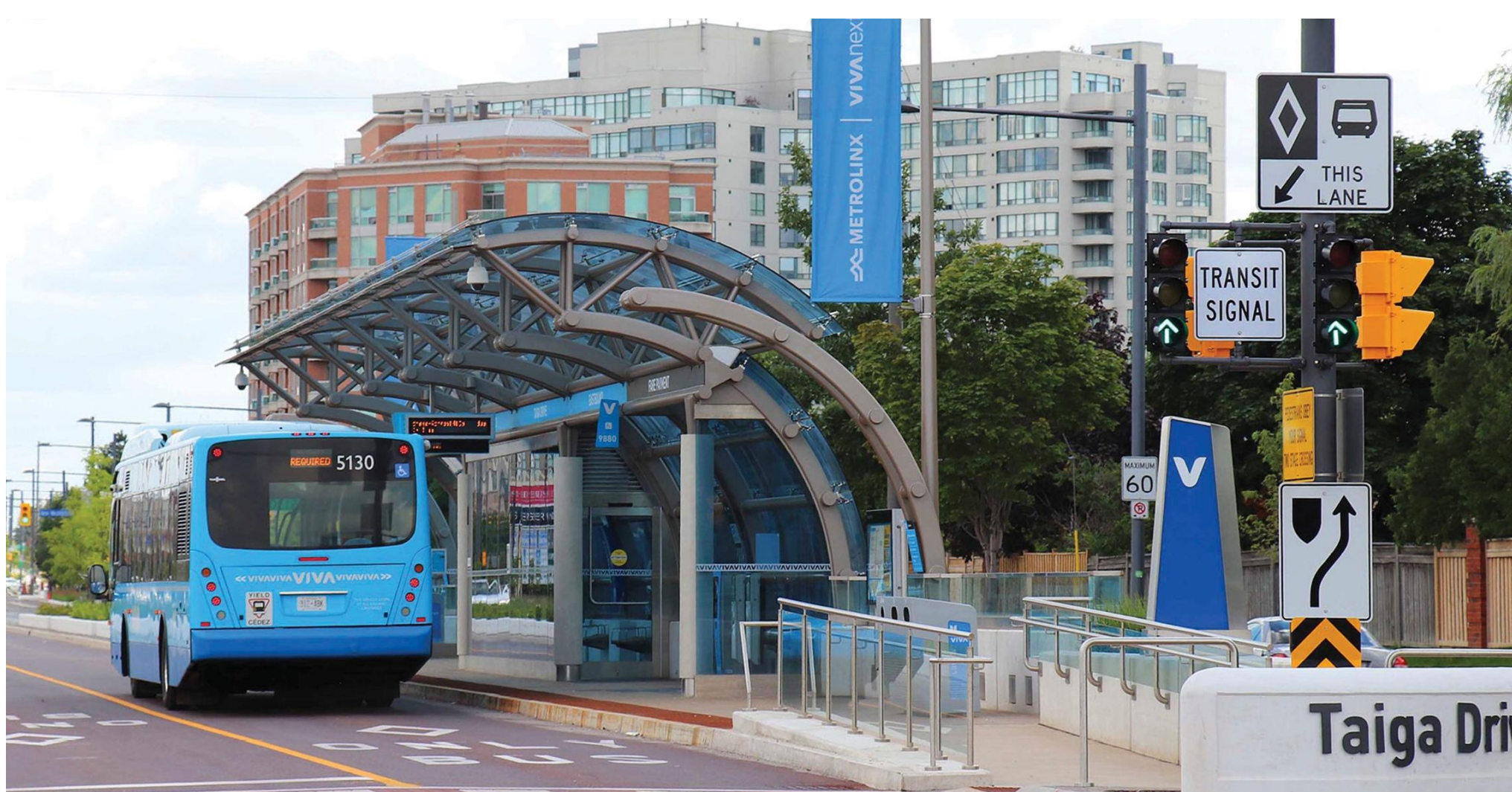
Example of an improved Arterial Street (Centre Street, Vaughan)
