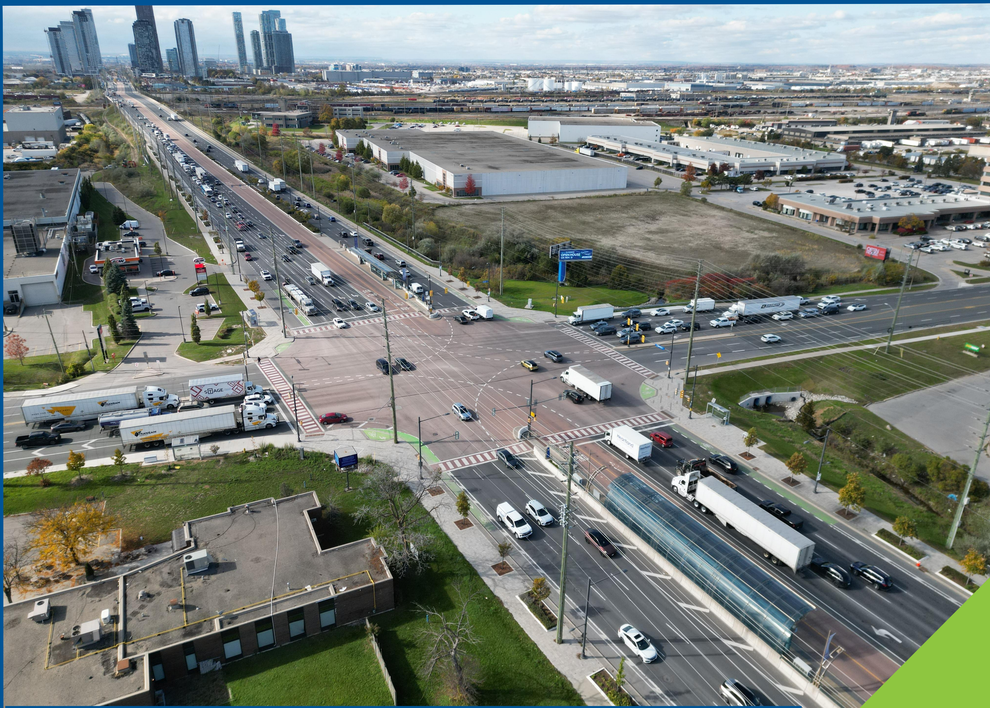
Looking west along Highway 7 towards the Vaughan Metropolitan Centre
