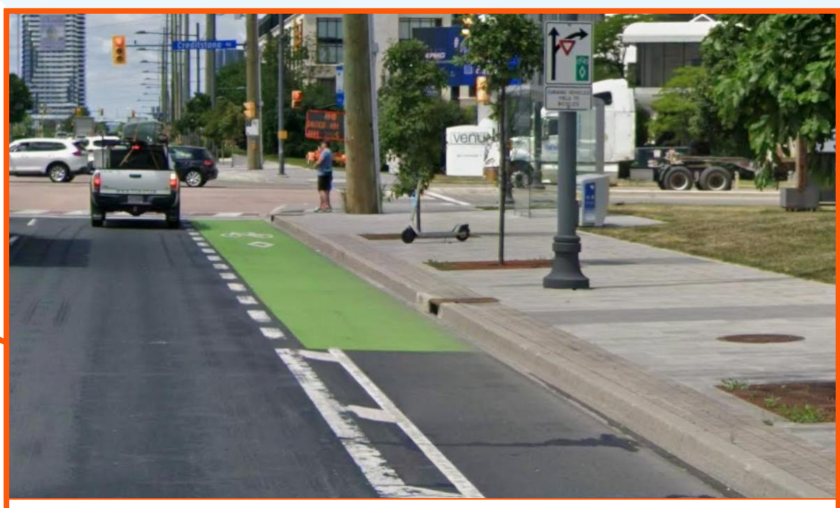
Painted bike lanes exist along portions of Highway 7 and Dufferin Street. Due to high vehicle speeds and volumes, they do not meet the all ages and abilities network standard.
