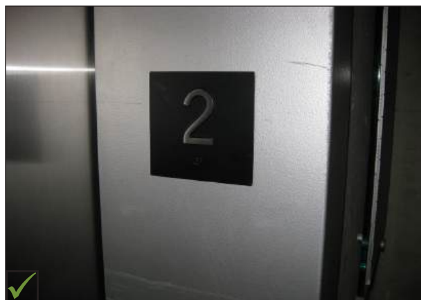
Tactile elevator car identification sign.
