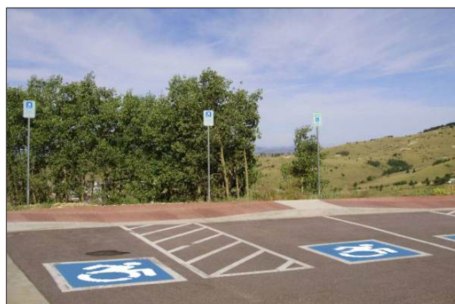
Accessible parking spaces and access aisle.
