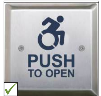
Large power door operator control, clearly marked with International Symbol of Accessibility.
