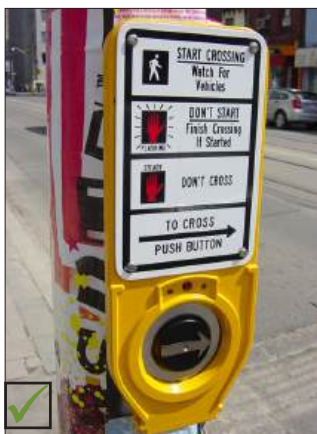
Typical APS actuation.
