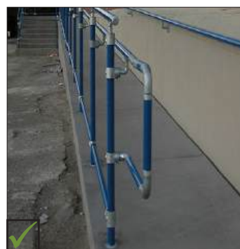
Figure 19b: Handrail Returns to Wall
