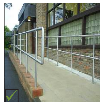
Figure 19c: Handrail Returns to Floor
