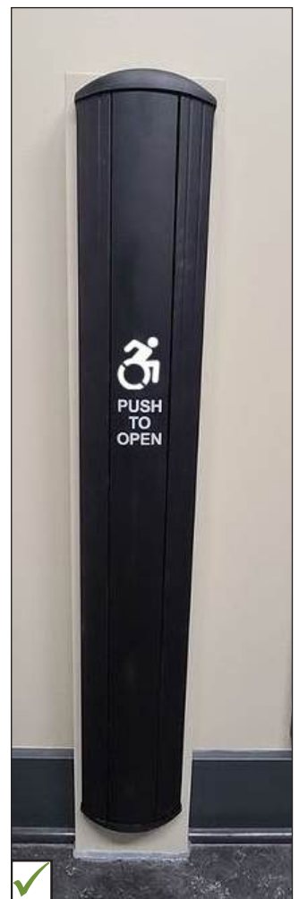
Long extended power door operator control can accommodate a wider range of users (e.g., can be operated by foot or foot rest).
