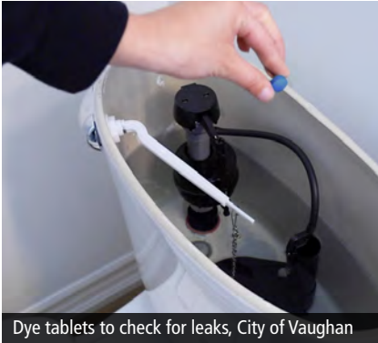
Dye tablets to check for leaks, City of Vaughan
