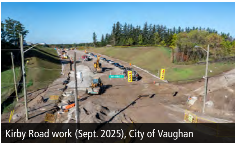
Kirby Road work (Sept. 2025), City of Vaughan
