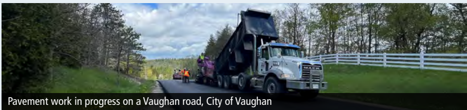
Pavement work in progress on a Vaughan road, City of Vaughan
