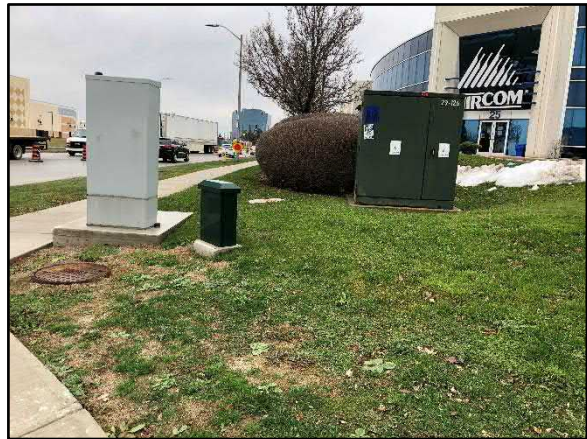
Image 60: Evidence of underground infrastructure under manicured boulevard. Note: access panel, man hole, transformer in foreground. Facing northwest.
