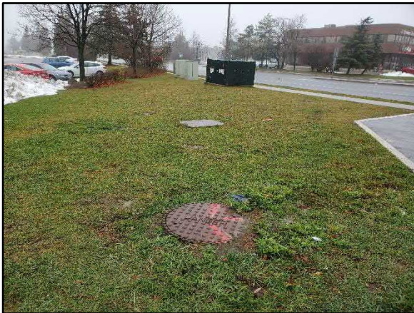
Image 47: Evidence of underground infrastructure under manicured boulevard. Note: man hole and access panel in foreground and transformer in background. Facing northeast.
