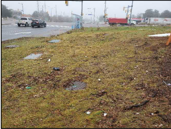
Image 45: Evidence of underground infrastructure under manicured boulevard. Note: man hole and access panels in foreground. Facing south.
