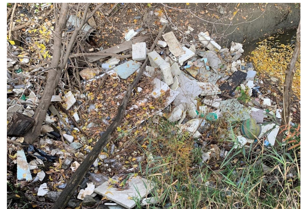
Photo 4: Garbage pile at culvert
