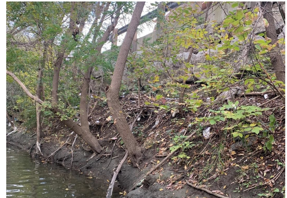
Photo 8: Armour stone supporting slope
