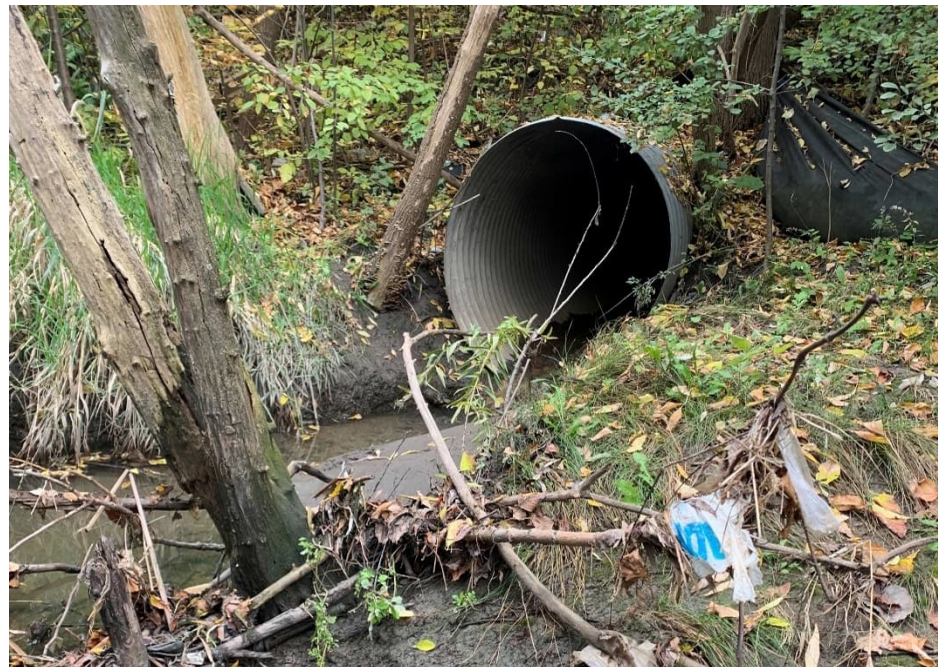
Photo 7: CSP culvert upstream of culvert
