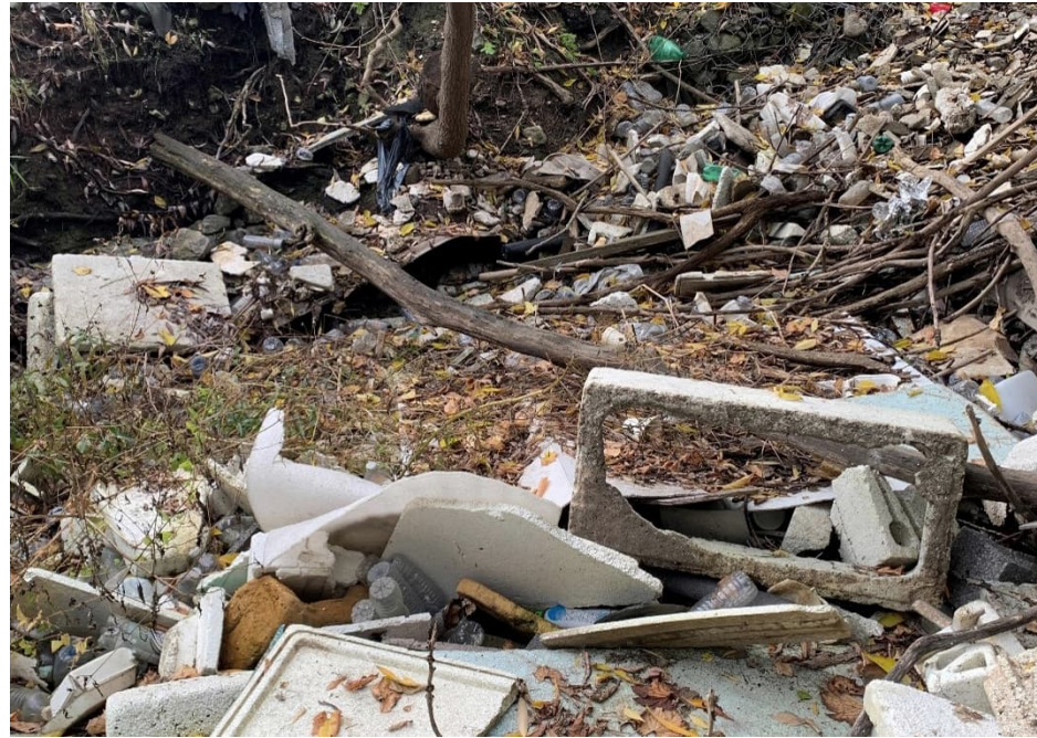
Photo 1: Culvert conveying creek south
