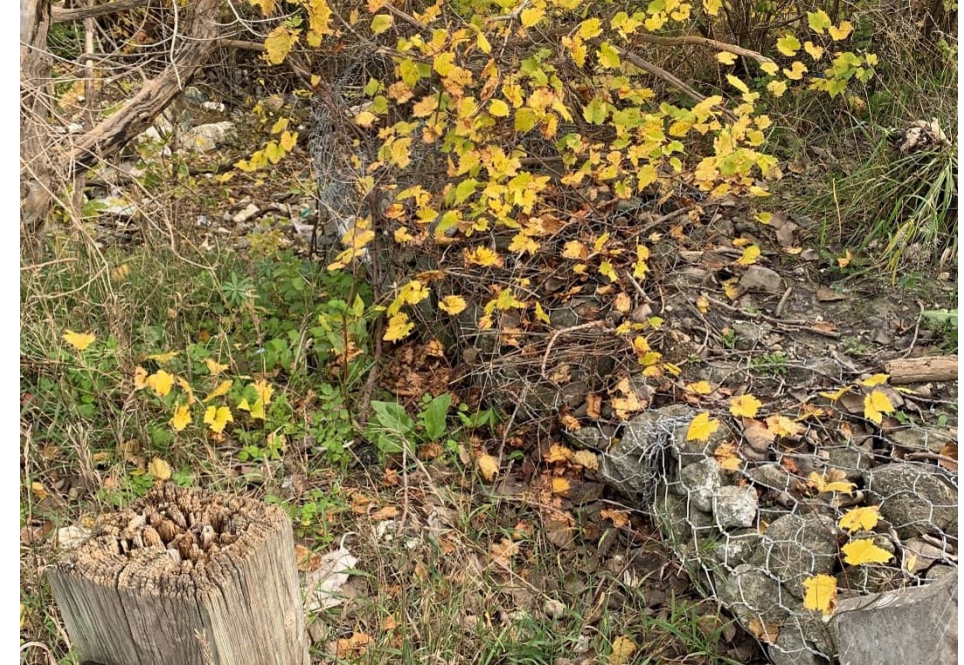
Photo 6: Gabion at crest of bank above culvert
