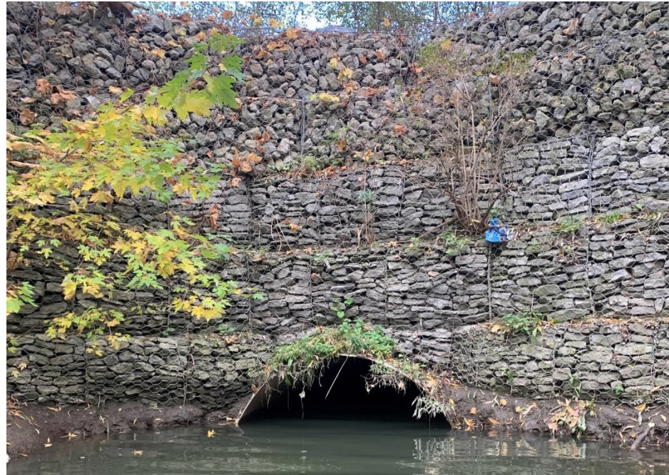
Photo 9: Culvert outlet into deep pool at base of gabion wall
