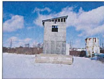
City of Vaughan's Existing Tower
