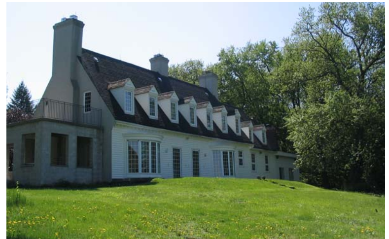
Huntington Road stud farm “summer house”
