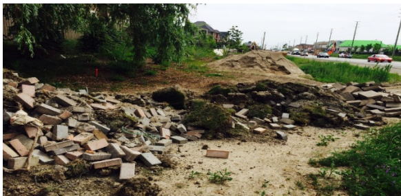
FIGURE 14 - EXAMPLE OF DUMPING
