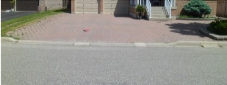
FIGURE 11 - EXAMPLE OF INCORRECT DRIVEWAY WIDENING
