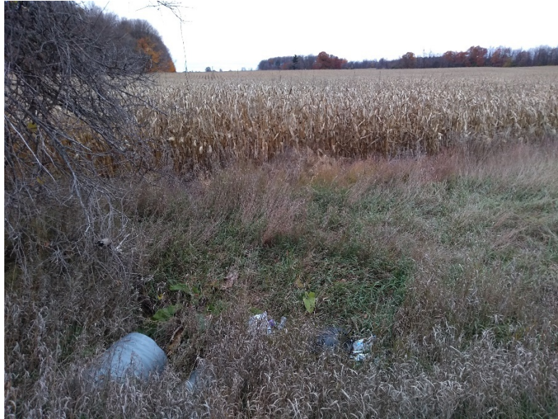
Figure 3 Looking north from the twin culverts.
