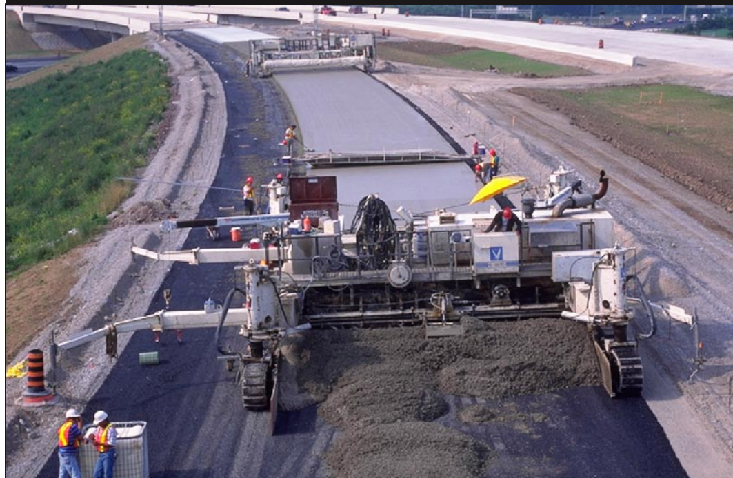
Fig. 4. Construction of 407 ETR.
