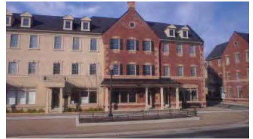
A new townhouse development in Maple.
