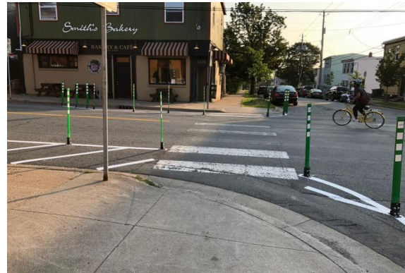
Temporary Curb Extension
