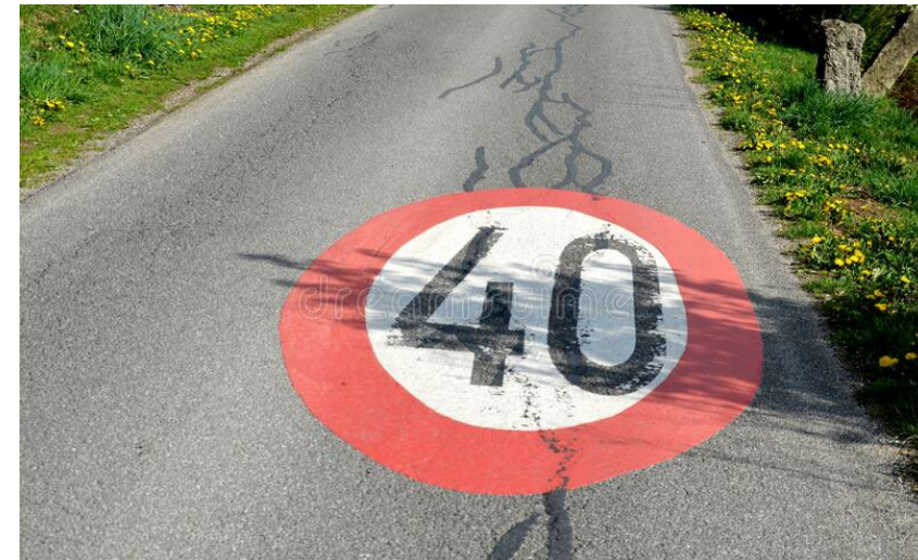
40 Km/H Pavement Marking
