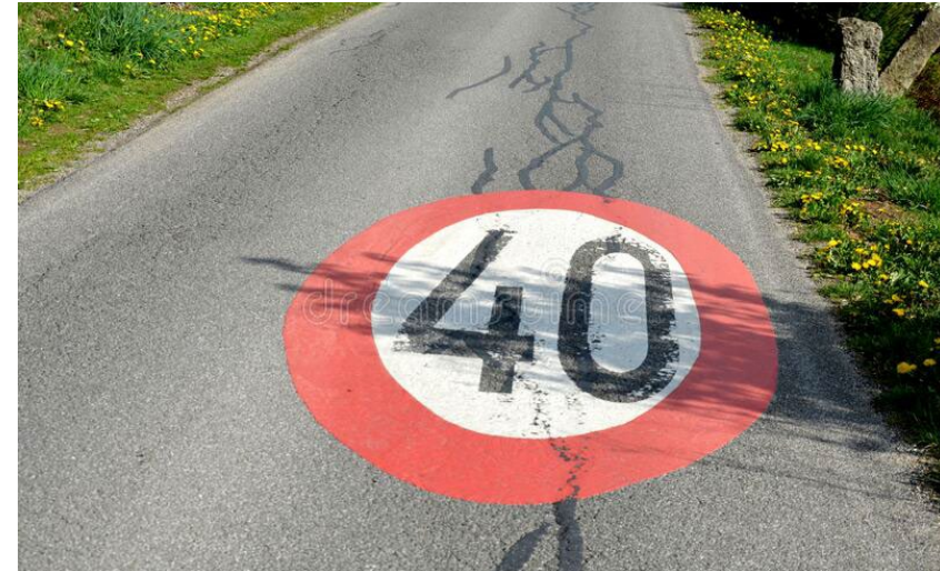
40 Km/H Pavement Marking
