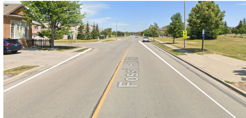
Edgelines to visually reduce road width
