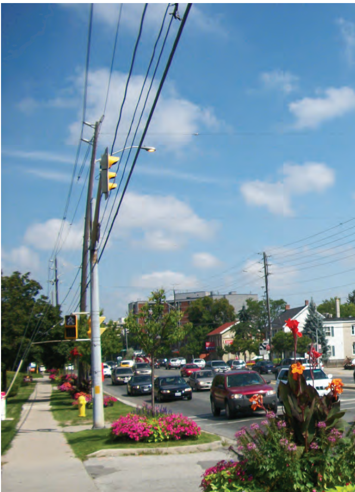
Street with Overhead Hydro Wires
