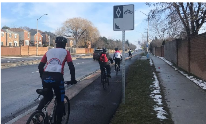
In-boulevard Cycle Track along Clark Avenue substantially constructed in 2020
