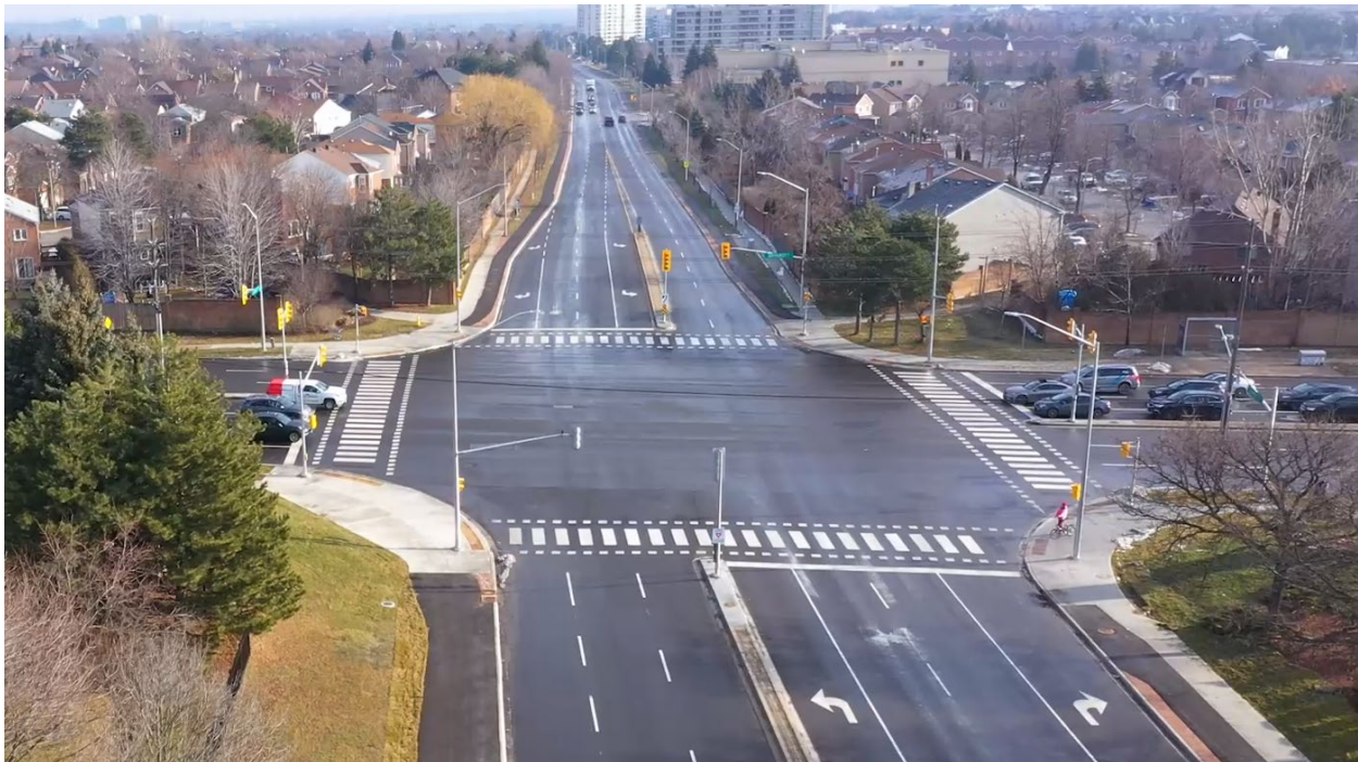
Example of standalone active transportation project – Cycle tracks along Clark Avenue at Bathurst Street substantially constructed (2020)
