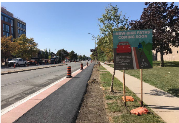
Cycle tracks under construction along Clark Avenue (2020)
