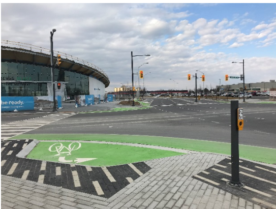
Bike Box at Millway Avenue and Applemill Road within the Vaughan Metropolitan Centre (VMC)
