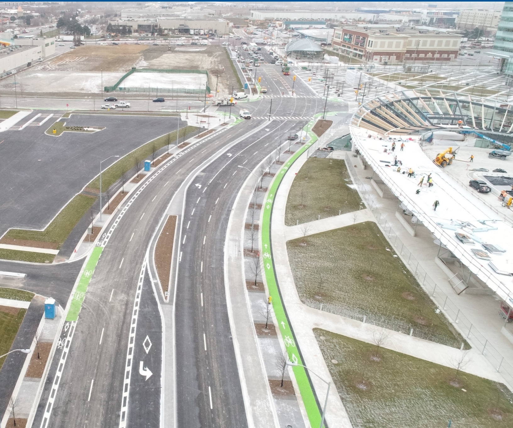
Wide sidewalks and cycling facilities along Millway Avenue in the Vaughan Metropolitan Centre (VMC)
