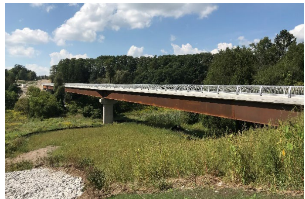
Purpleville Creek pedestrian bridge at Pine Valley Drive and Teston Road
