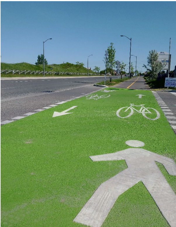
In-boulevard multi-use pathway along McNaughton Road East
