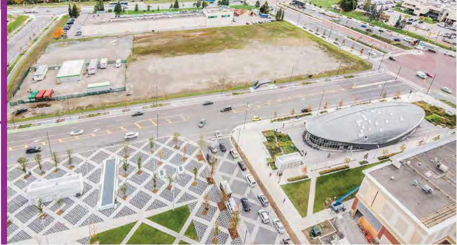
Millway Promenade - North Of Highway 7
