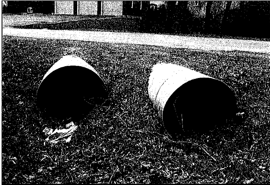
Photo 37 Outlet of 2 x 800 mm CSP crossing culvert C6 on Brooke St. north of Arnold Ave. Culvert is in good condition
