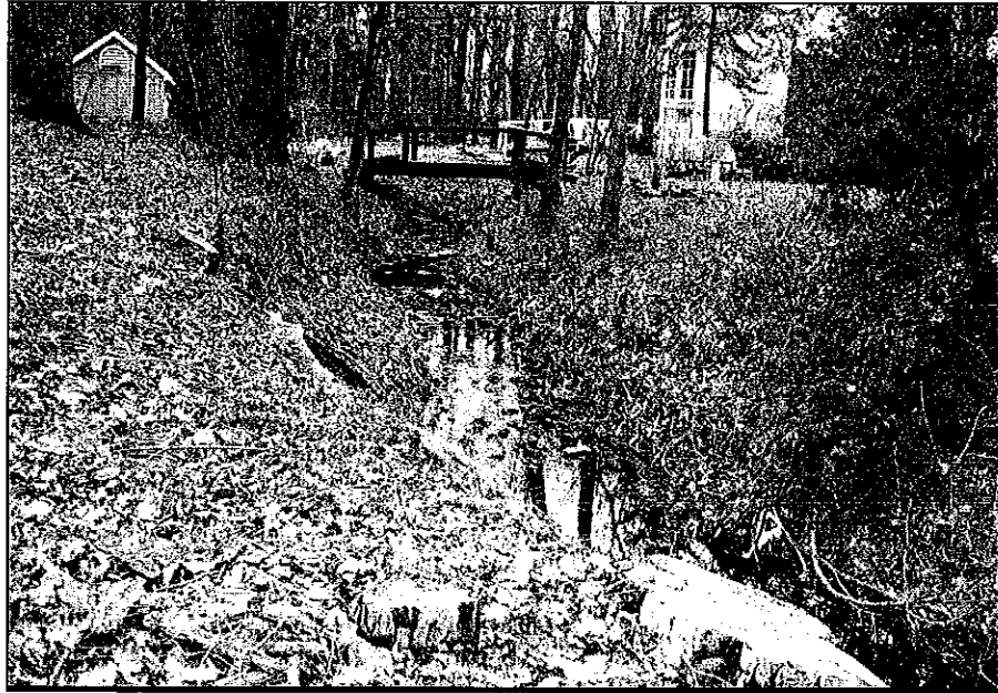
Photo 15 Drainage Course #1, upstream of Culvert C17
