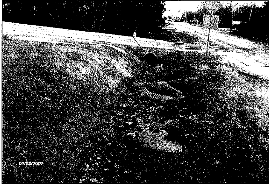
Photo 25 600 mm CSP driveway culvert D1 at the driveway of 132 Arnold Ave. Culvert is undersized
