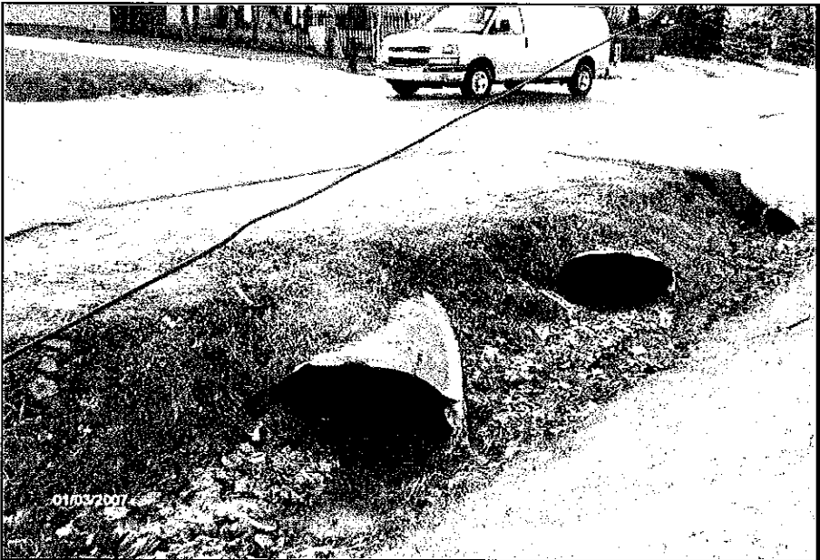
Photo 24 Outlet of 700x1100 mm CSPA crossing culvert C1 on Arnold Ave., west of Charles St. minor deformation
