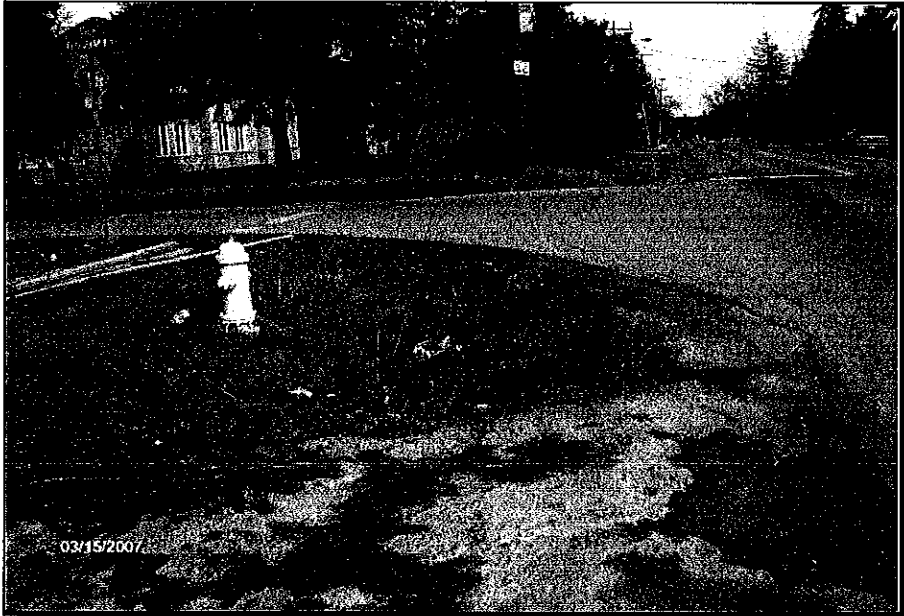
Photo 41 Inlet of side road culvert on the north side of Arnold Ave. at Clarkhaven St. Culvert inlet is buried due to construction activity
