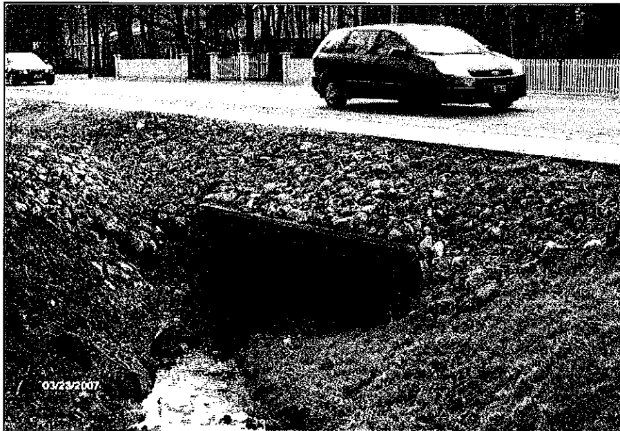
Photo 22 1200x2500 mm crossing culvert C16 under Centre st. east of Donna Mae Cr.
