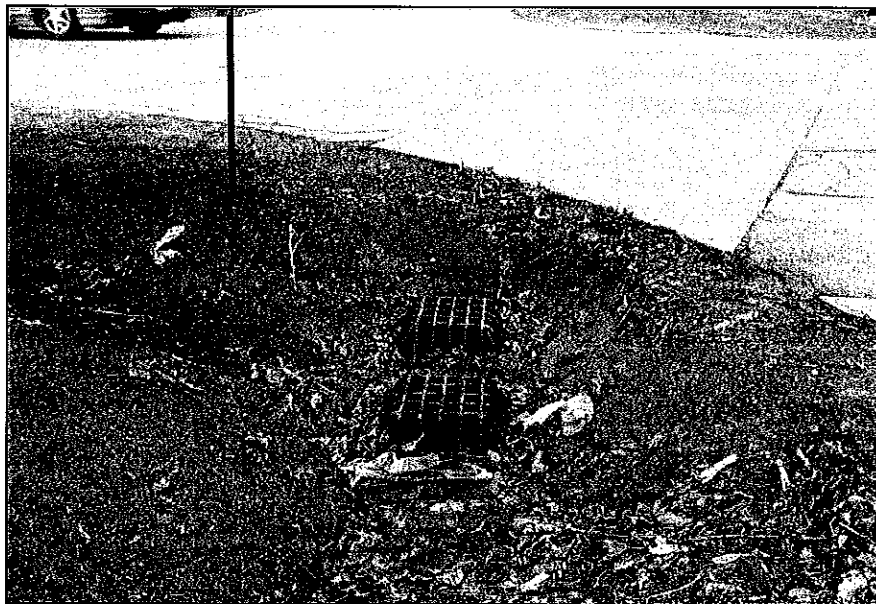
Photo 53 Twin Ditch Inlet DICB 2 at the south west corner of Brooke St. and Arnold Ave. Twin ditch inlets and the connecting 375 mm pipe is undersized.
