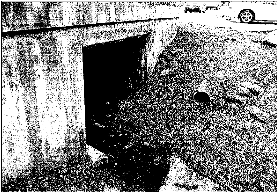
Photo 14 Downstream of Culvert C17
