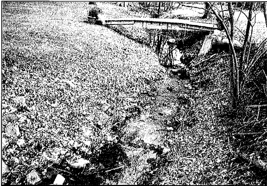
Photo 16 Drainage Course #1, downstream of Culvert C17
