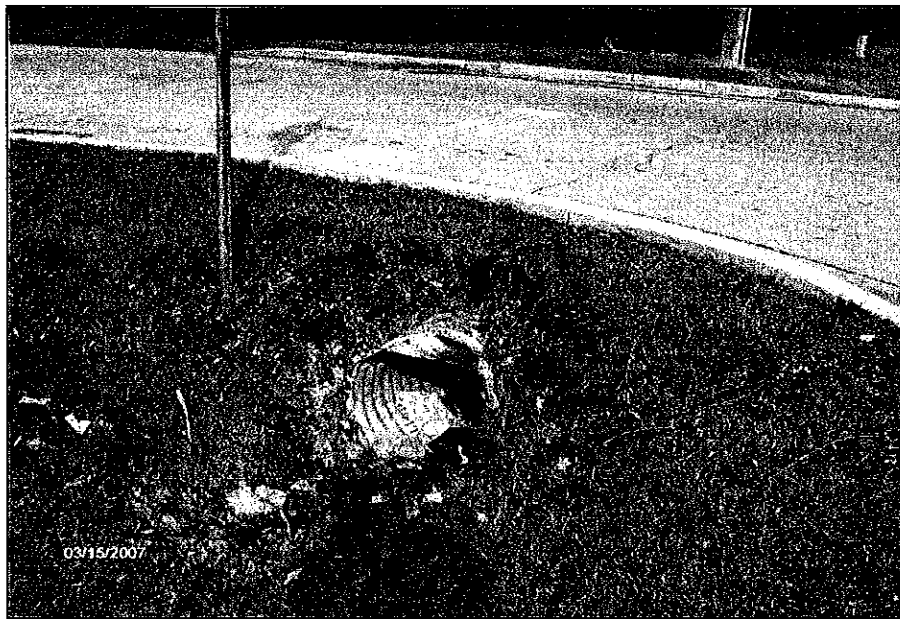
Photo 6 675 mm CSP side road culvert under Erica Rd. north of Centre St. capture runoff from the west side ditch and convey it to the Oakbank Pond
