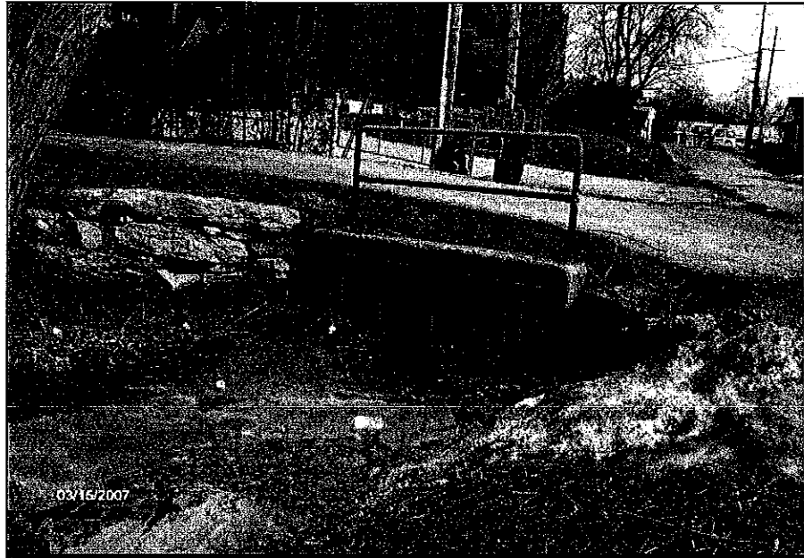
Photo 19 Upstream of Culvert C19
