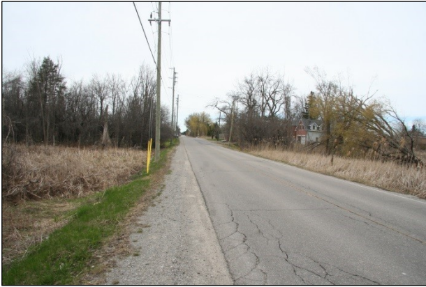
Plate 21: North view along Huntington Road showing wet areas on both west and east sides of roadway.
