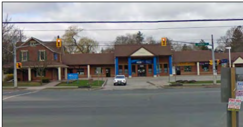
Auto Oriented Retail Plaza Integrated with Older Residential Dwelling (Google Earth Image)
