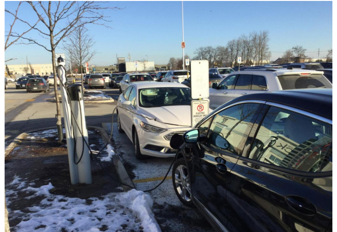
Example: EV Charging Stations
