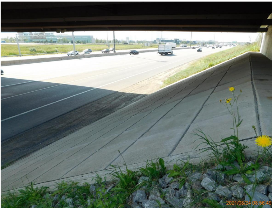
46 West Concrete Slope Protection
