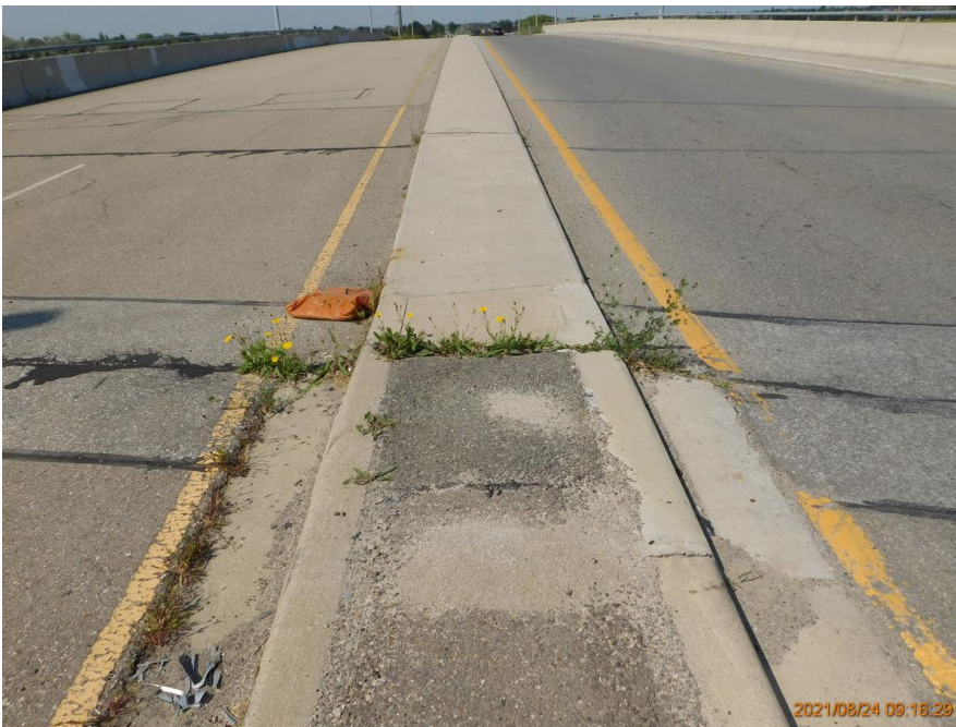
24 Center Median at East Approach, Looking West
