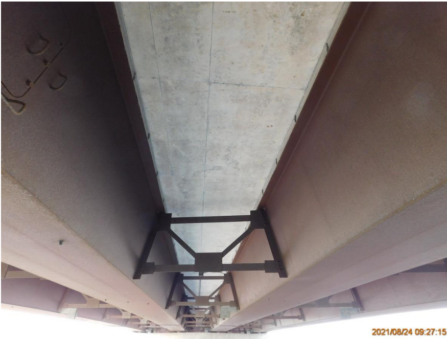
13 Interior Soffit and Girders at East Abutment, Looking West
