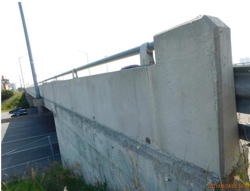
20 North Exterior Barrier Wall, Looking East
