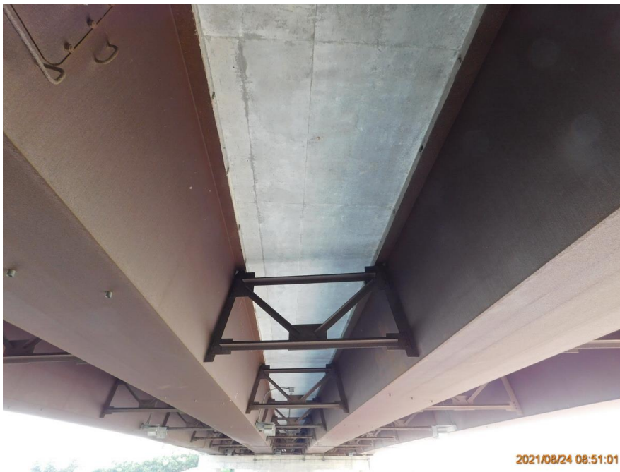
12 Interior Soffit and Girders at West Abutment, Looking East
