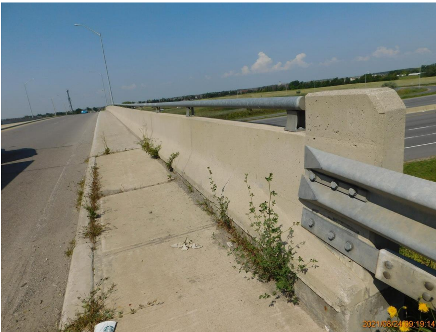
22 North Interior Barrier Wall and Sidewalk, Looking West
