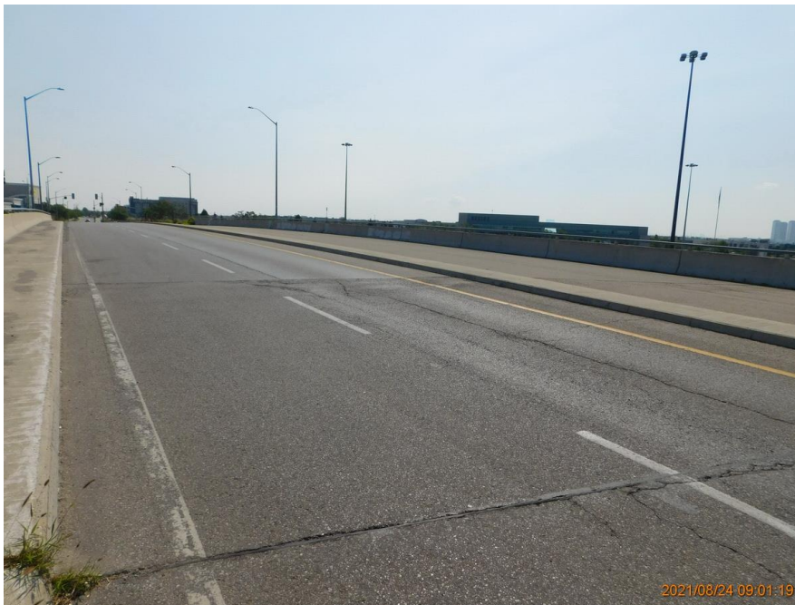
04 Bridge Deck From Northwest Corner
